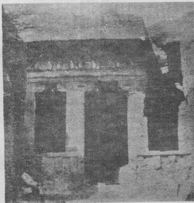
Fig. 1. Cave No. 6, The Barī Kachahri, General View.
