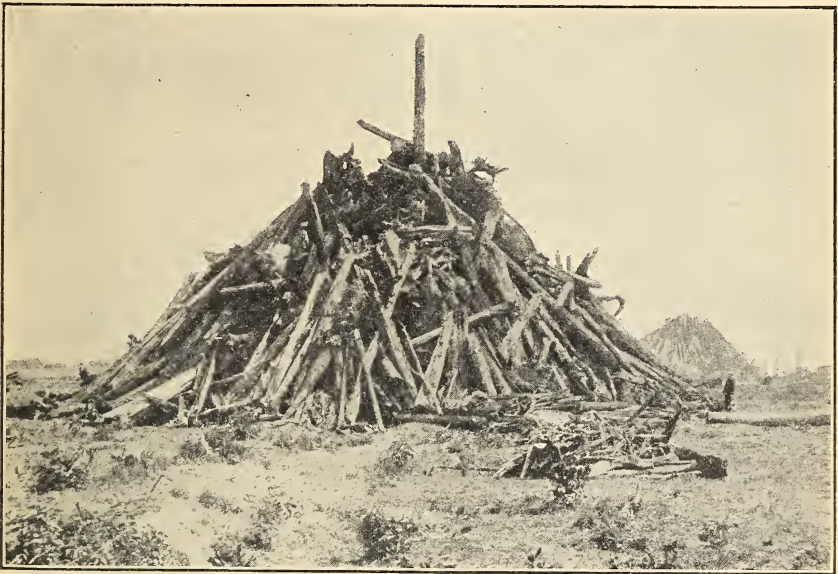
FIG. 6.—Stumps piled around gin pole in clearing with donkey engine.
