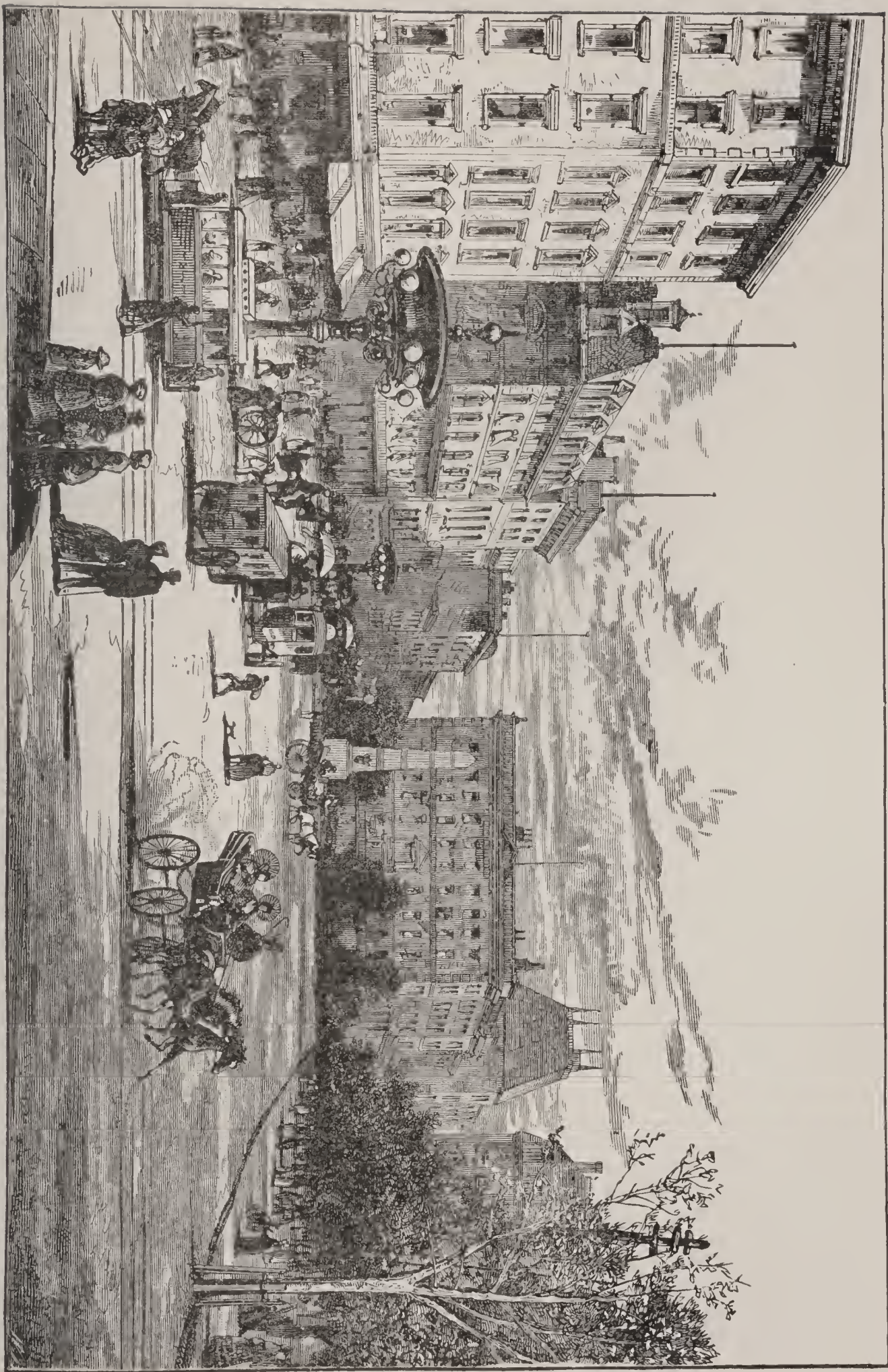
New York.—Broadway and Opening of Fifth Avenue at Madison Square.
