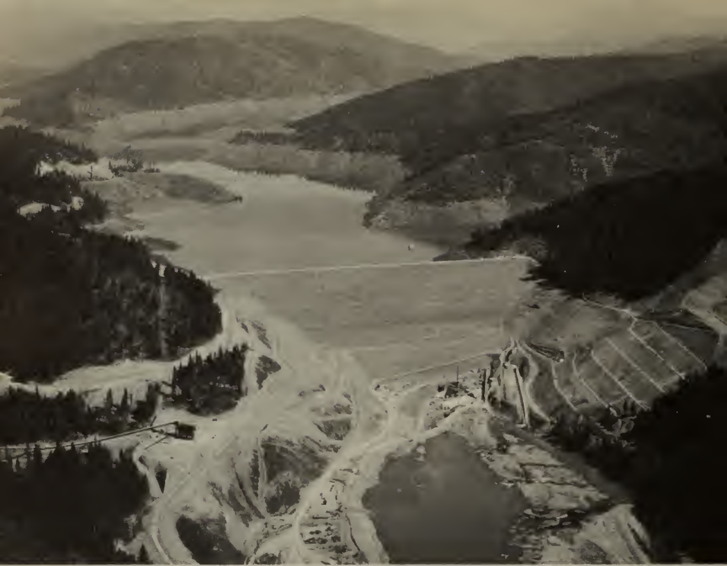
Trinity Dam, Bureau of Reclamation's largest earth-filled structure, backs up the Trinity River in northern California.
