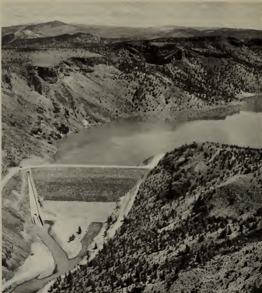
Prineville Dam on the Crooked River in Oregon stands completed.
