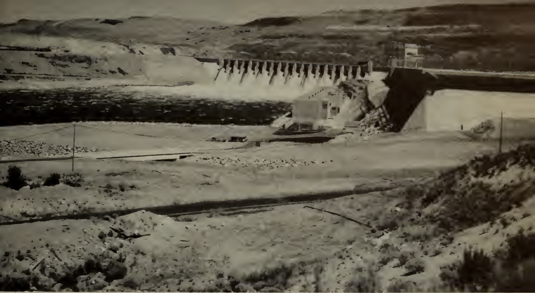
Chief Joseph Dam, one of the recently completed mid-Columbia projects supplies power for central and northwest Washington loads of Bonneville Power Administration.
