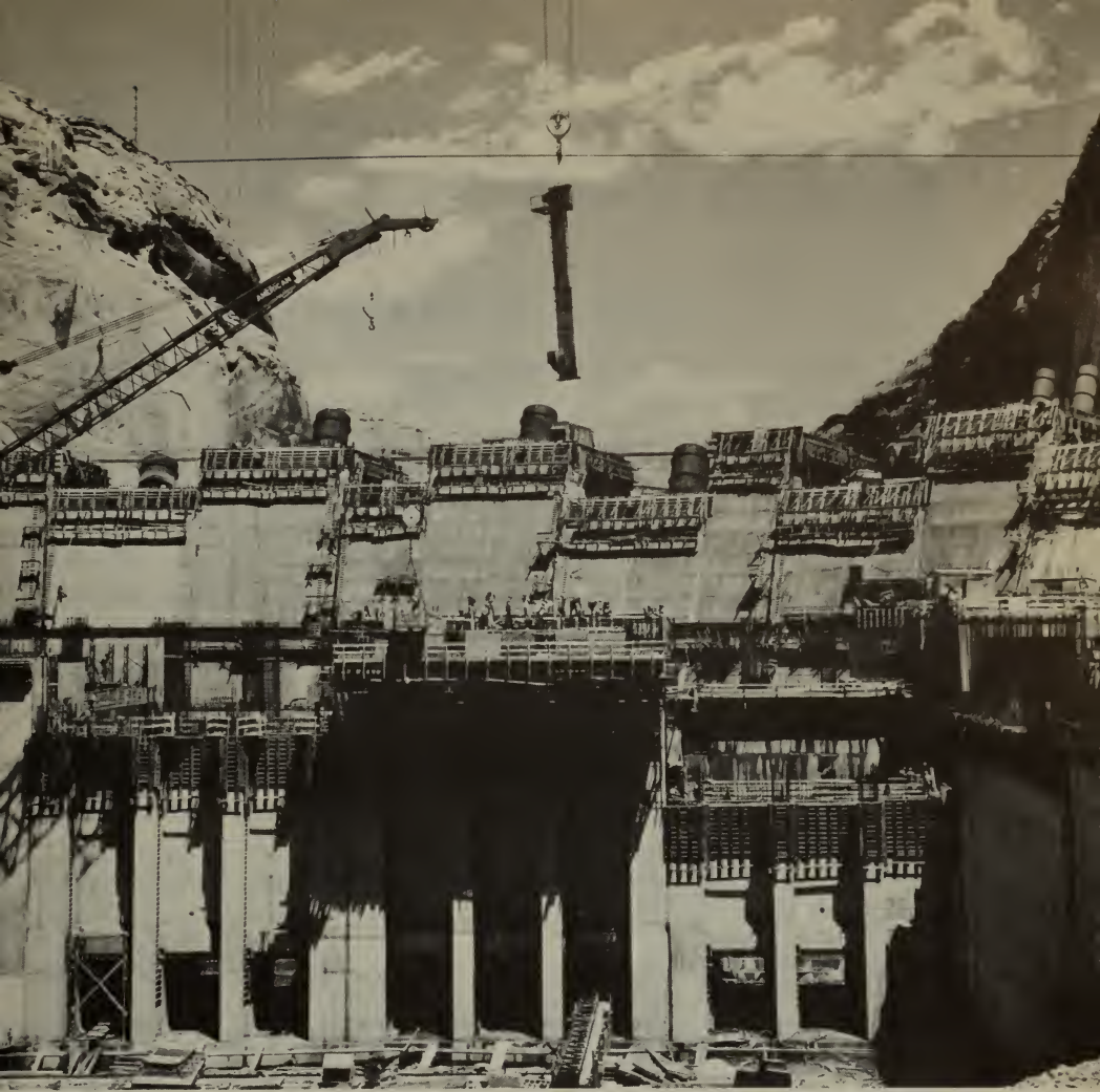
Glen Canyon Dam in Arizona, major Colorado River storage project unit, climbs toward its designed height of 710 feet.
