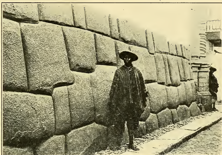
FIG. 41. Inca wall, Cuzco, built of augite diorite porphyry.
