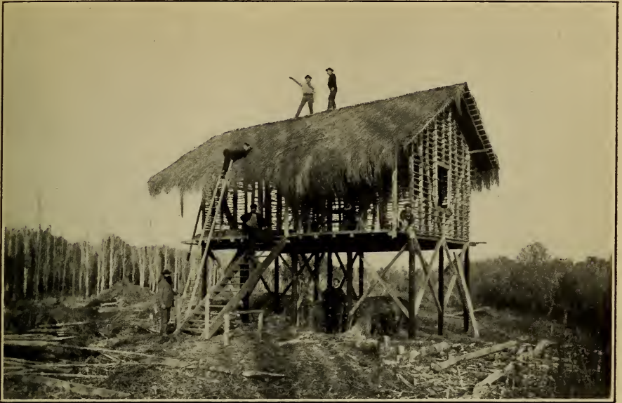
Building a House in Argentina, near Buenos Aires, where the river overflows its margins periodically. All the trees in view were planted.
