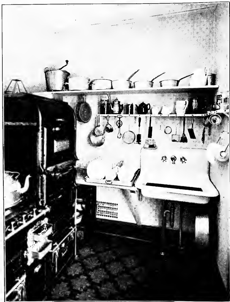
KITCHENETTE WITH GAS-RANGE.
