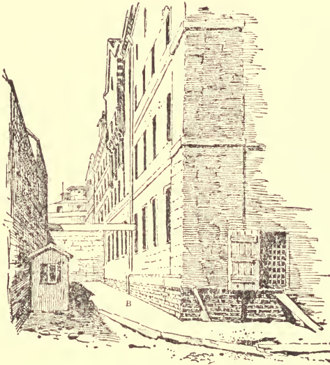
EXTERIOR OF THE PRISON. B—EXIT FROM TUNNEL.
