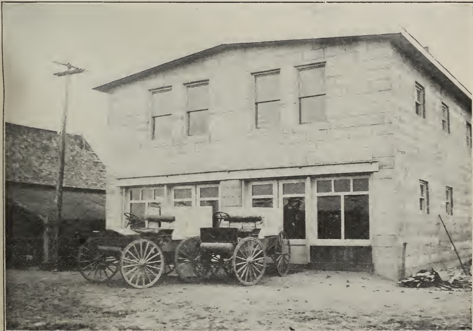
D. C. Polhemus' new building for a workshop, extracting-house, etc., and his two International auto wagons which he uses to carry the combs to and from the apiaries.
