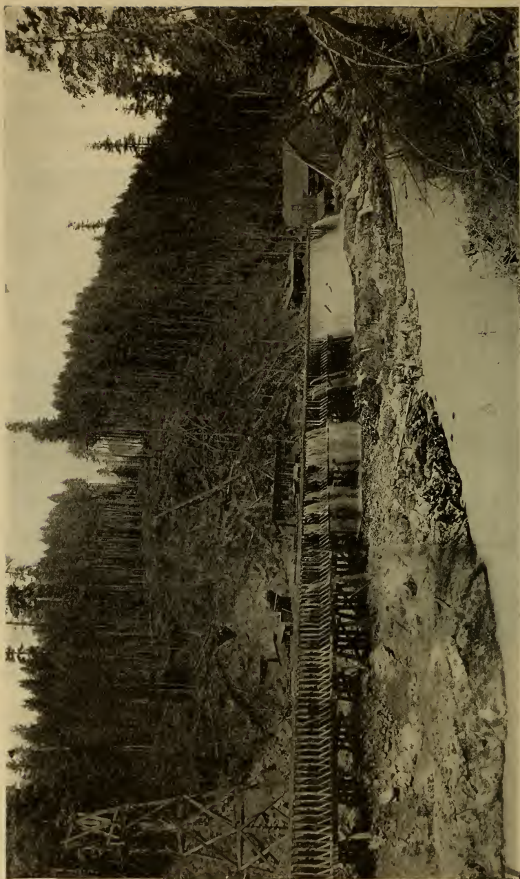
FIG. 11. View showing power-house, portal, and part of flume, Nisqually tunnel, Alder, Washington.
