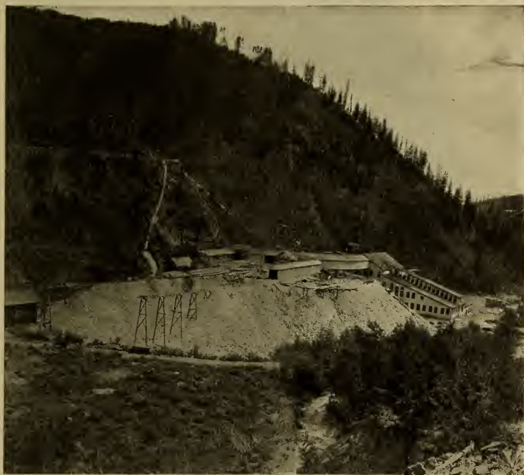
FIG. 10. View showing end of flume, mill, dump, and other surface features at Carter tunnel.
