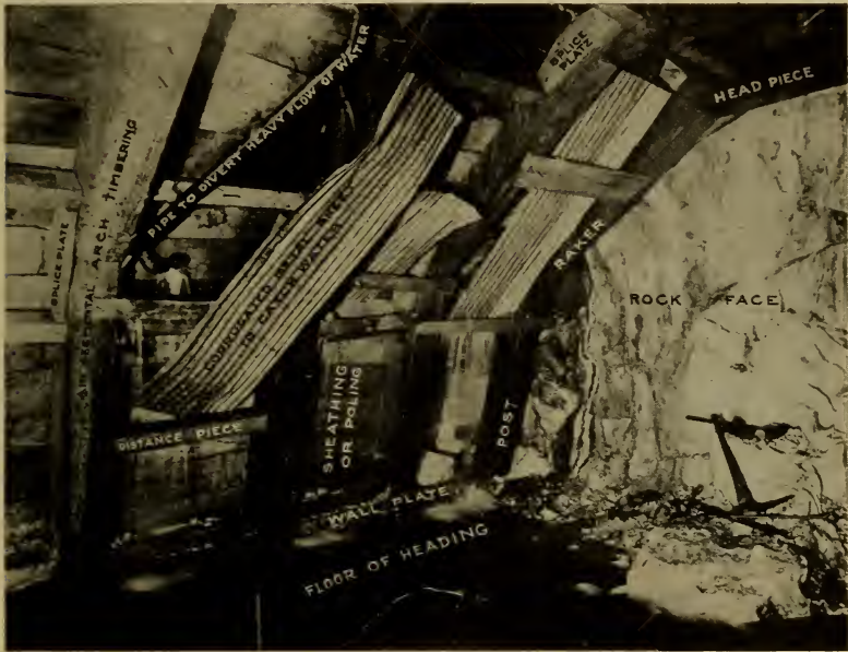
FIG. 106. American system of timbering Astoria gas tunnel, New York.
