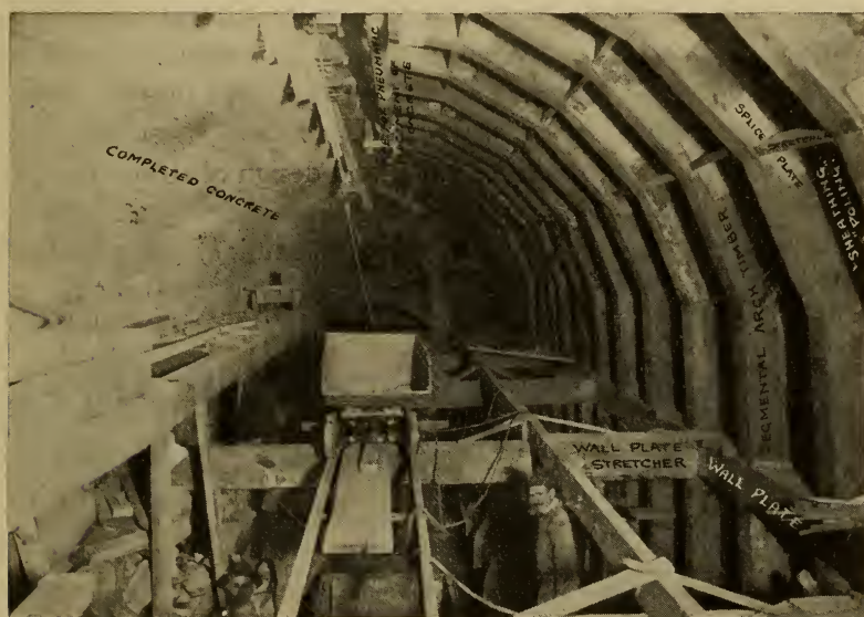
FIG. 81. Tunnel timbering. American system.
