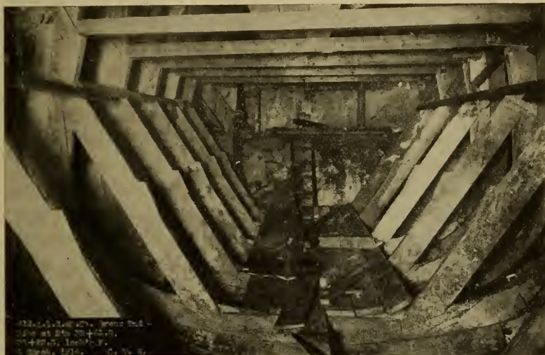
FIG. 111. Wooden forms for invert and sidewalls, Astoria gas tunnel, New York.
