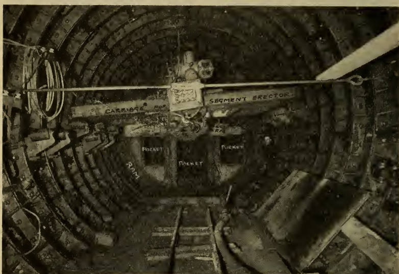
FIG. 117. Shield of Hudson & Manhattan Railroad under Hudson River, New York.
