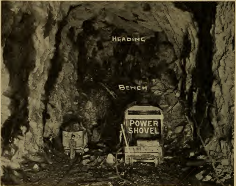
FIG. 89. Power shovel in rock tunnel.
