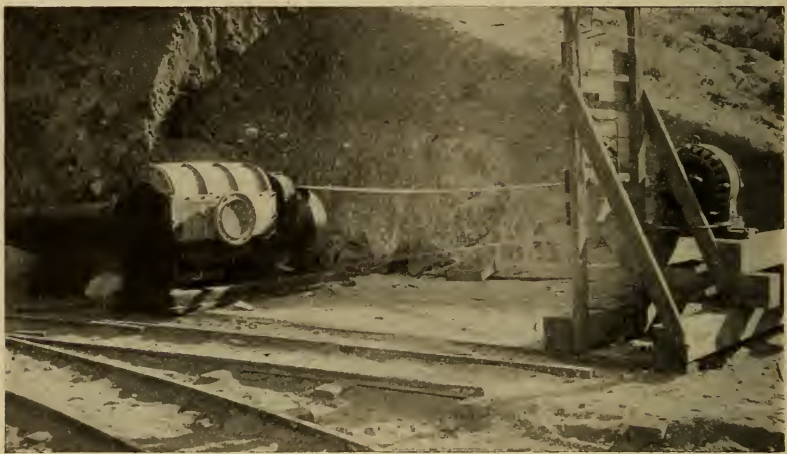
FIG. 26. Ventilating blower used on Los Angeles Aqueduct.
