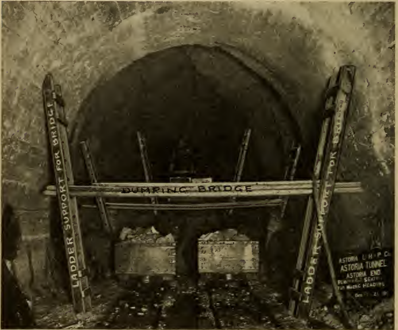
FIG. 99. Removable scaffold for mucking heading. Astoria gas tunnel, New York.
