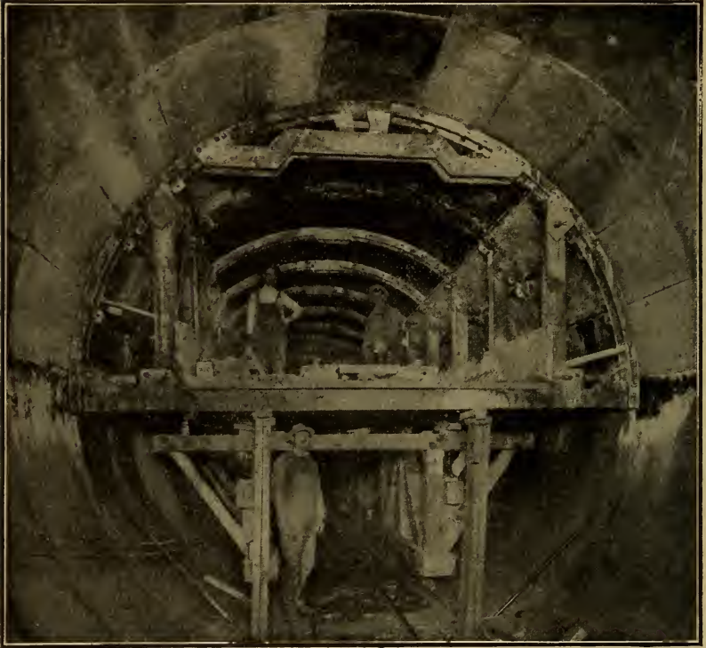
FIG. 112. Collapsible steel forms for tunnel arch lining.
