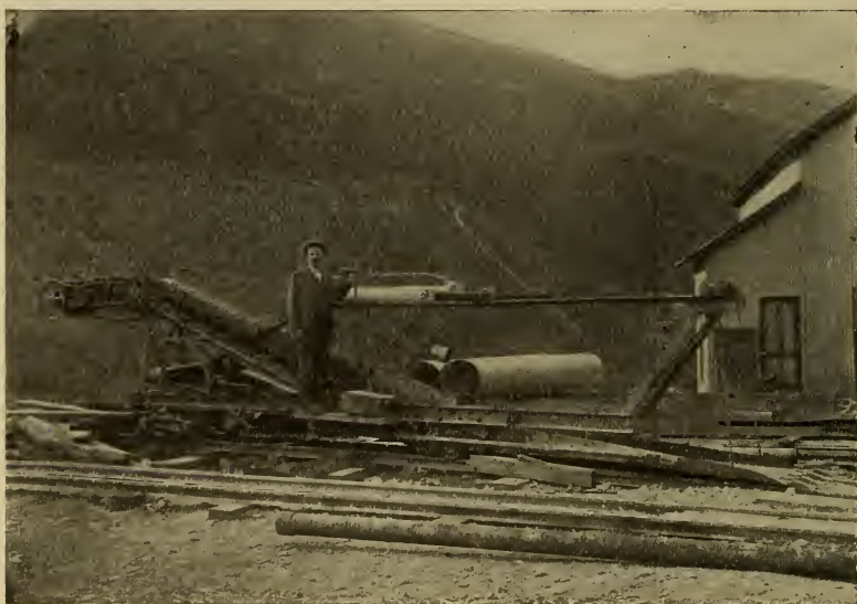
FIG. 54. "Mucking machine" at the Hummingbird tunnel, Burke, Idaho.
