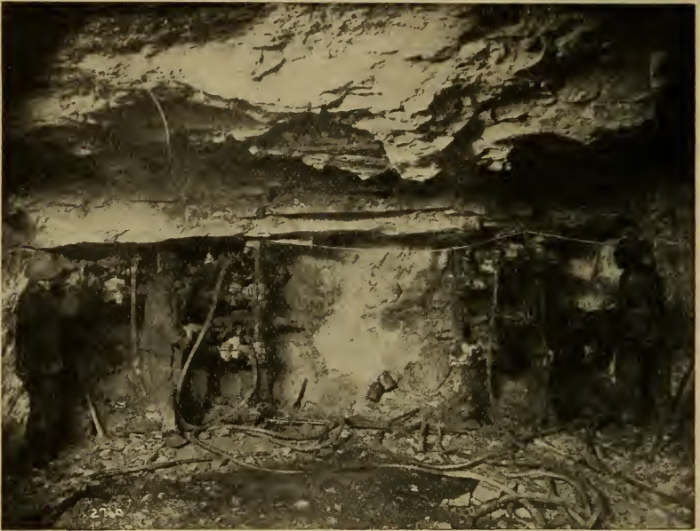
FIG. 4. Driving a modern tunnel with machine-drills.
