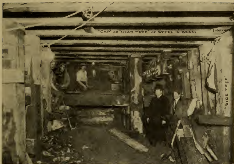
FIG. 109. Use of needle beam in heading.
