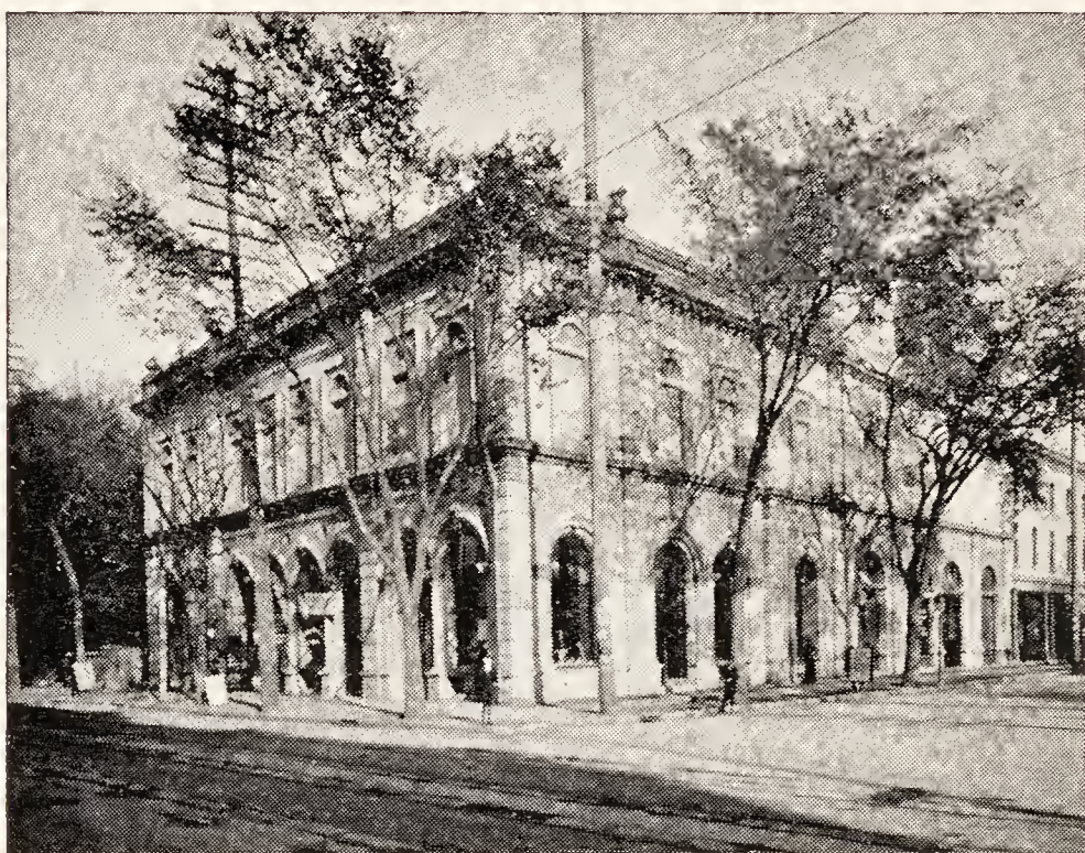
THE ART ASSOCIATION BUILDING, MONTREAL.
