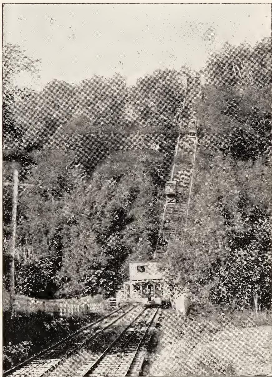
ELEVATOR ON THE EASTERN SLOPE OF MOUNT ROYAL.
