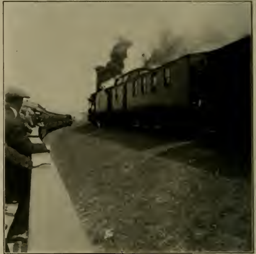
Observation Train Running Beside Demonstration Train of M. & L. Booster
