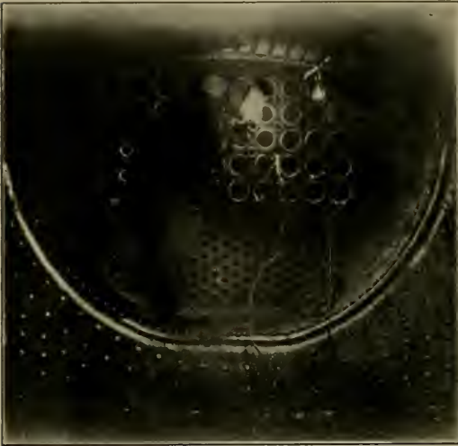
Fig. 3 Shows Firebox With Electric Welding Operator at Work
