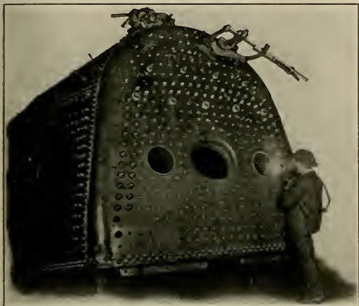
Fig. 5 Shows Method of Electrically Welding Openings in Back Head of a Firebox
