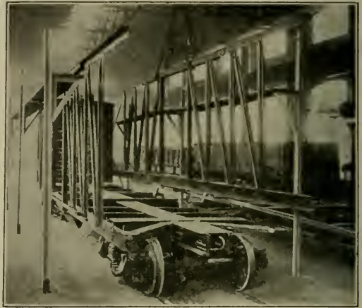
Placing the Side Frames in Position
