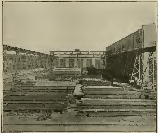
Storage Yard Along Front of Steel-Car Shop
