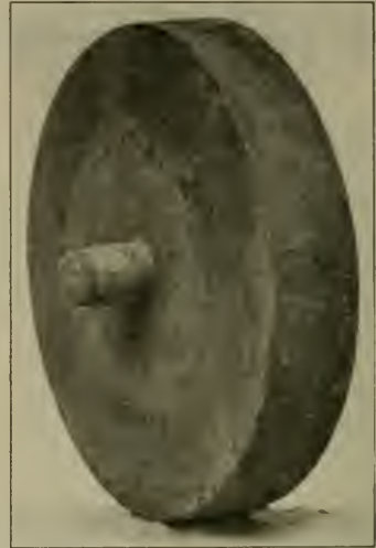
STEEL DISK MADE IN McCONWAY CASTING MACHINE
