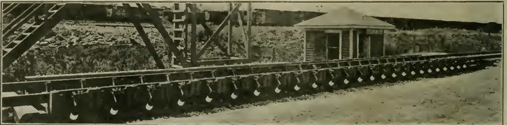
The Otheograph. Installation of 25 Units Under the Tracks at Erie, Pa.
