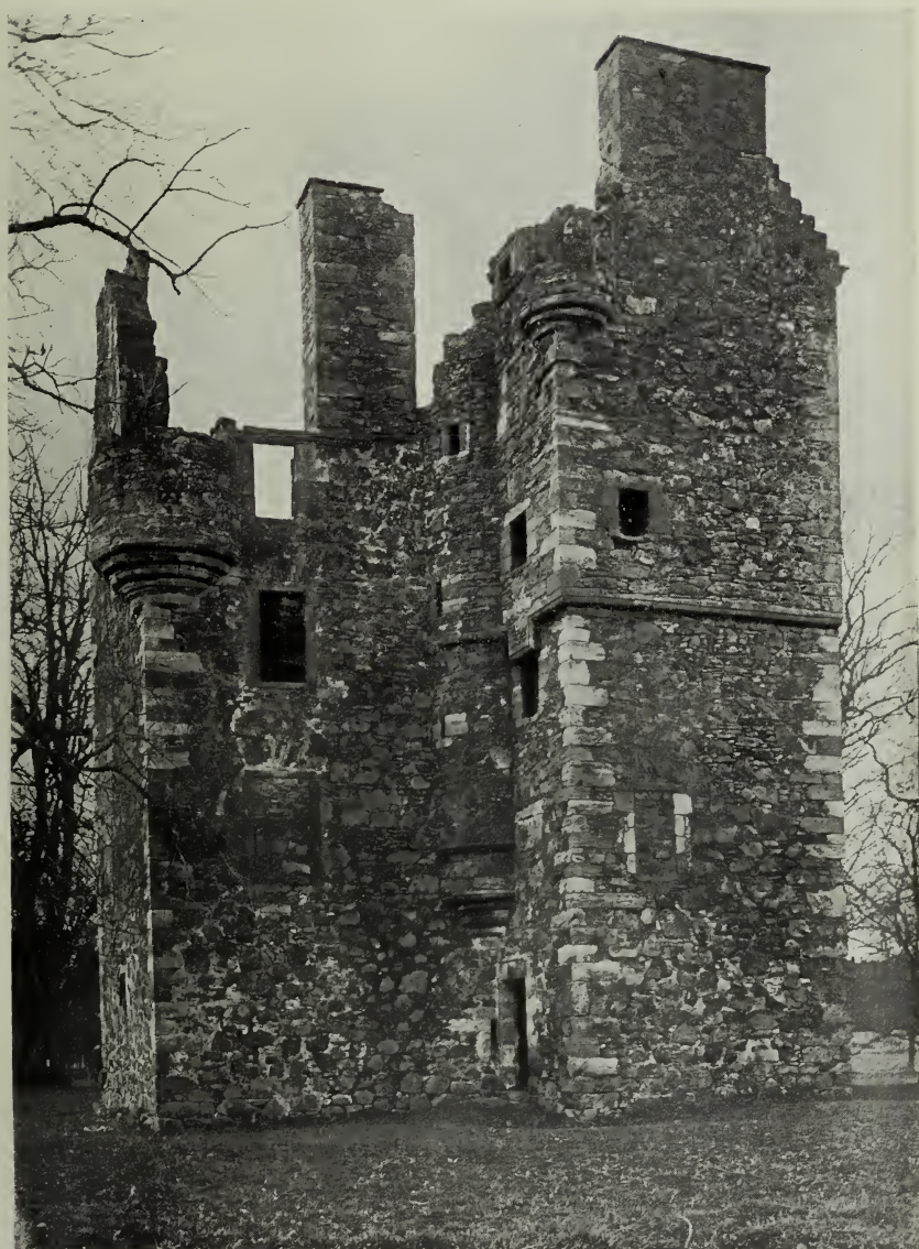
FIG. 84.—Greenknowe Tower from the South-east (No. 165).
