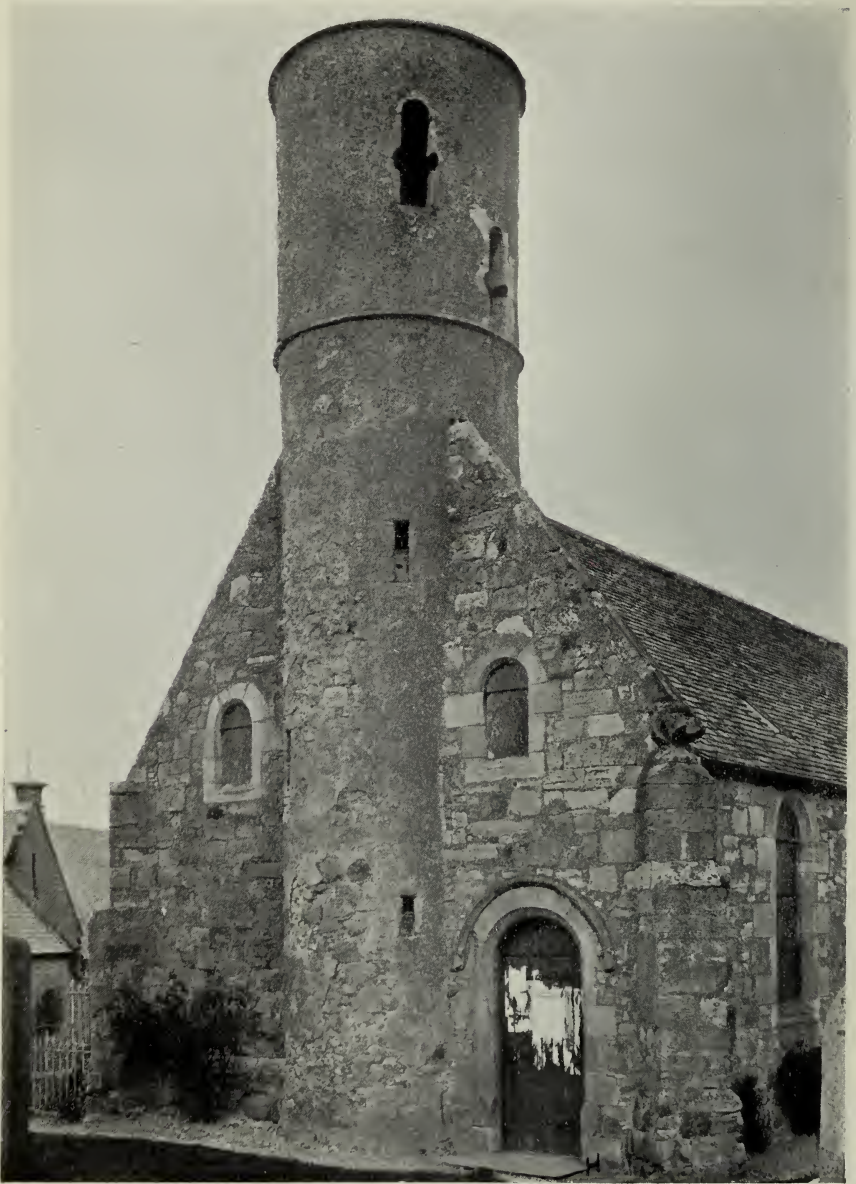
FIG. 18.—Cockburnspath Church : Tower (No. 45).
