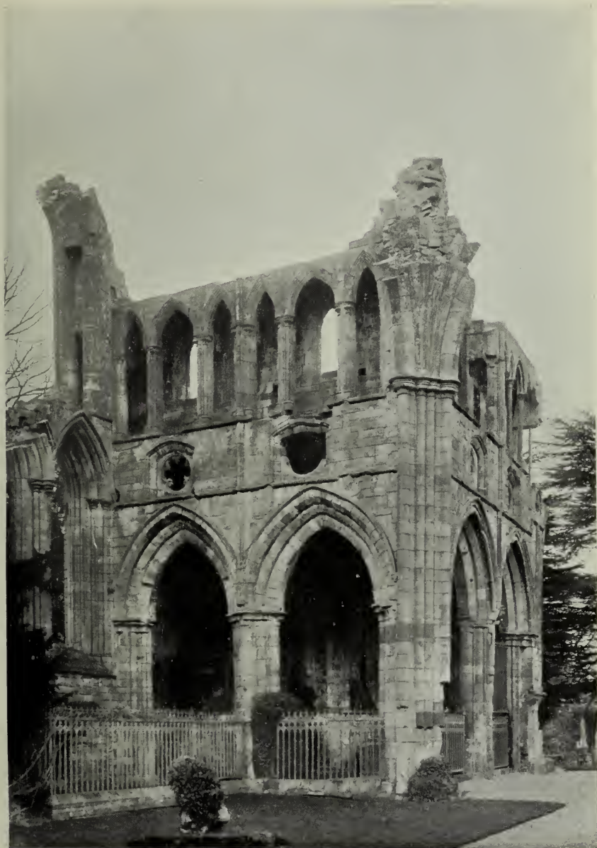
FIG. 125.—North Transept, Dryburgh Abbey (No. 258).
