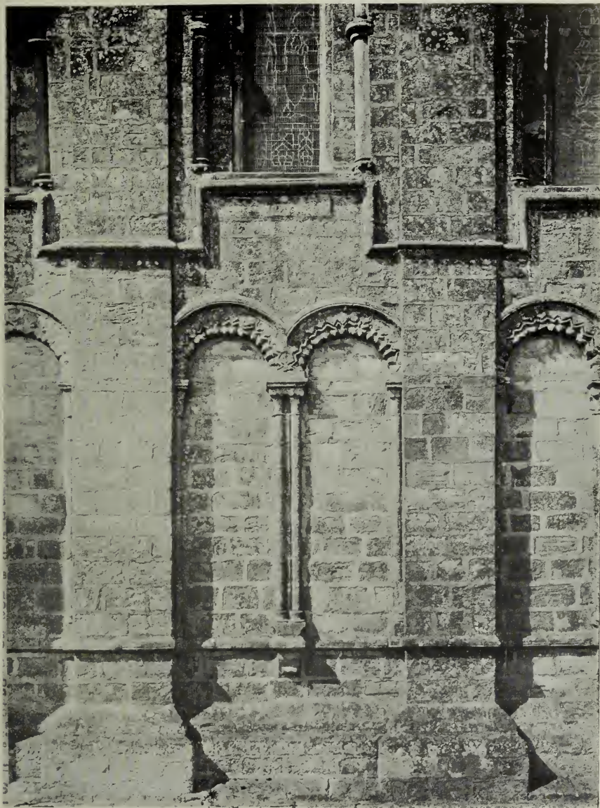
FIG. 38.—Detail of Wall Arcade, east end, Coldingham Priory (No. 74).
