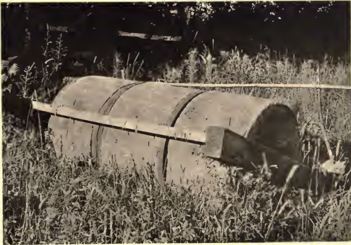
66. A HOME-MADE, THREE-SECTION WOODEN ROLLER
