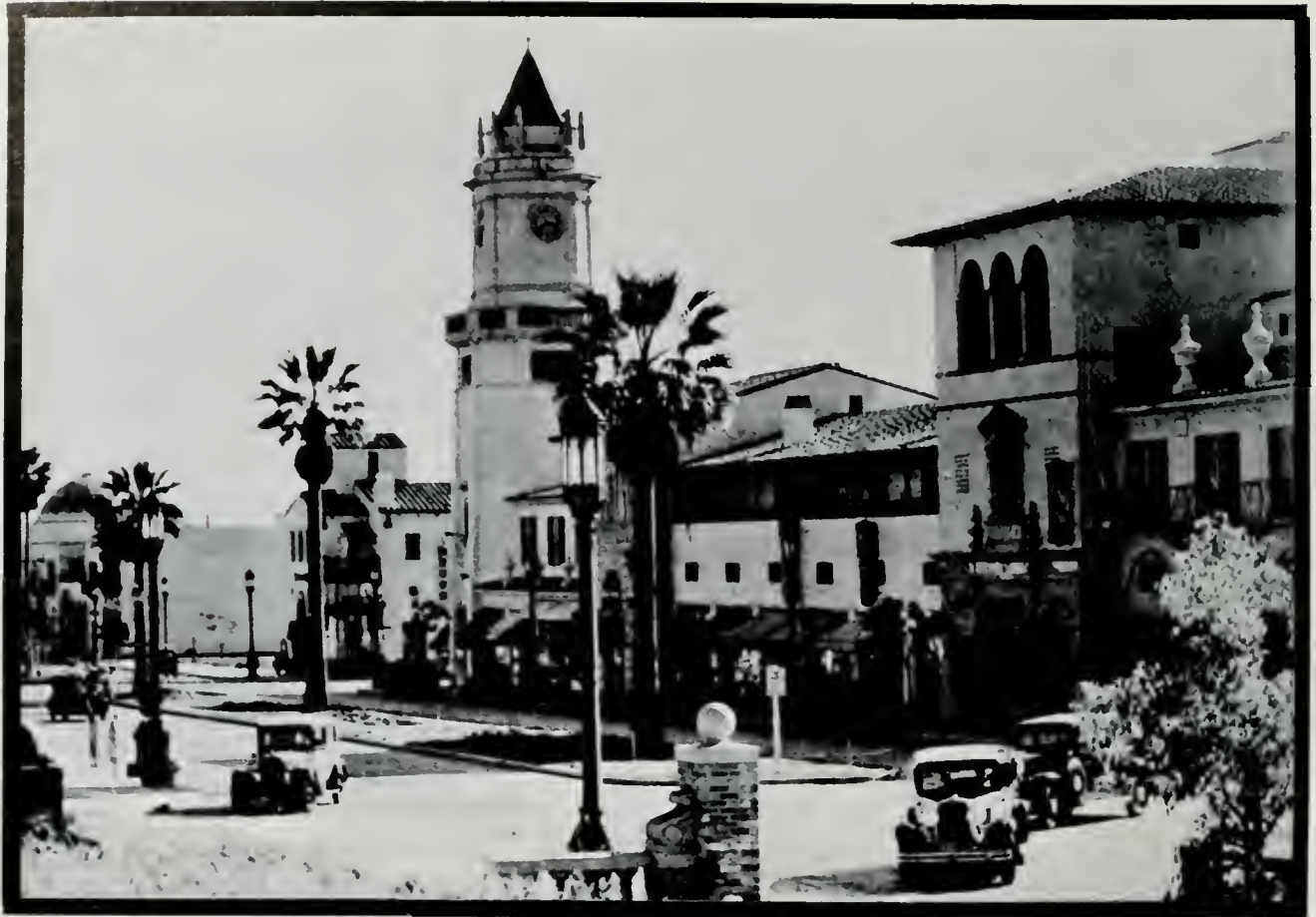
But by 1929 Westwood village merchants and residents were welcoming the arrival of the Southern Branch.
