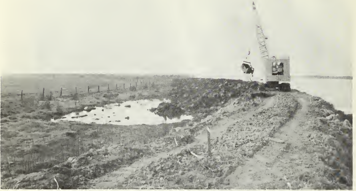
Photo 4. Dragline used for constructing and repairing levees and ditches.
