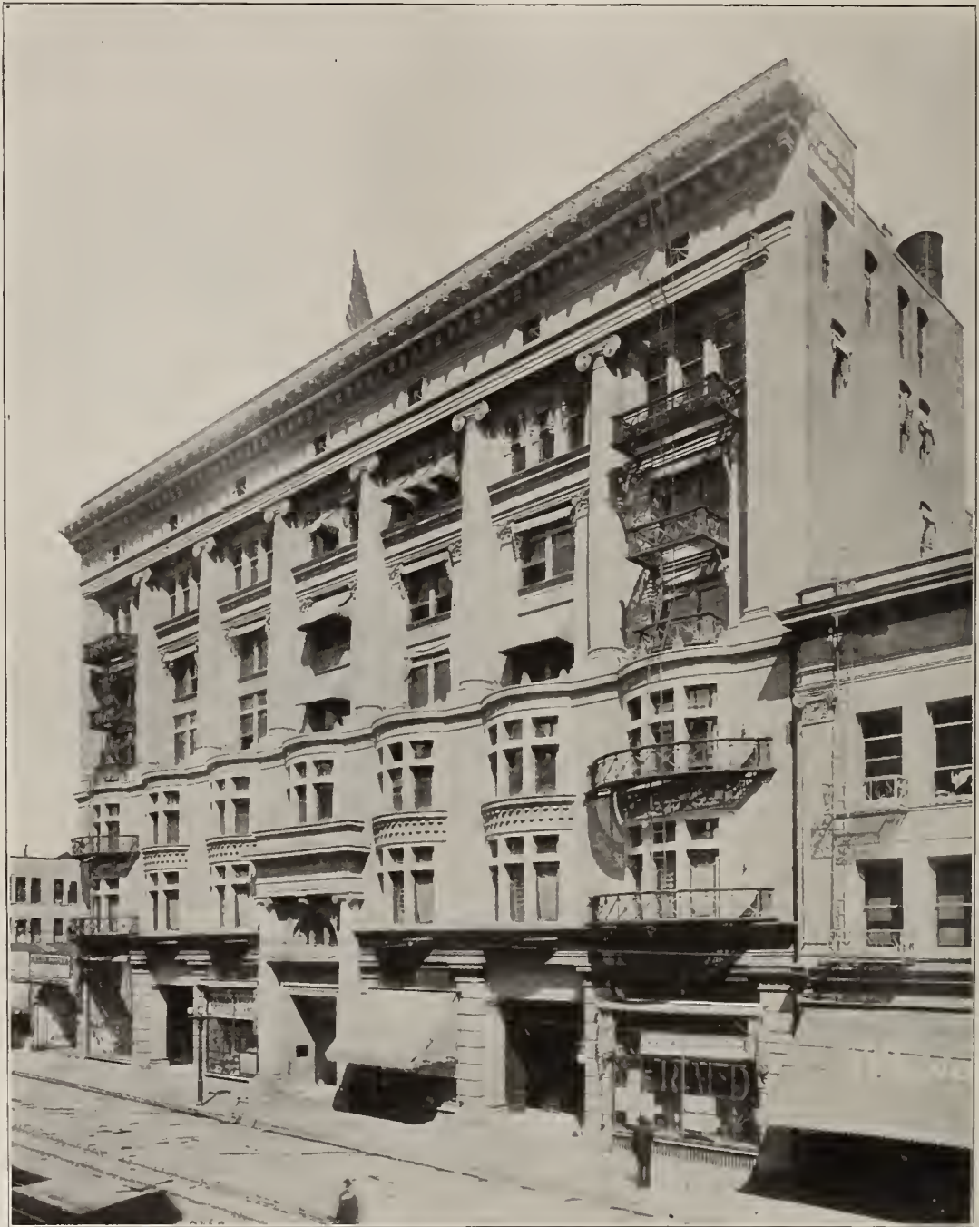
CHAMBER OF COMMERCE BUILDING, LOS ANGELES, CALIF.
