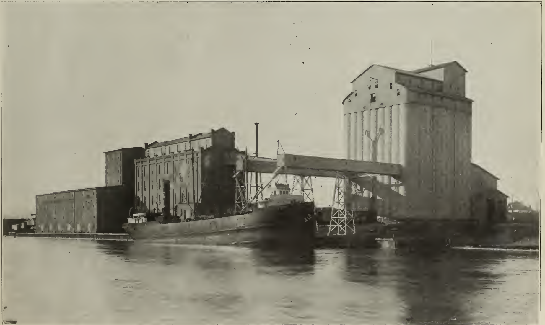
THE NEW STEEL GRAIN ELEVATOR OF THE OGILVIE FLOUR MILLS COMPANY, LIMITED, FORT WILLIAM, ONT. Macdonald Engineering Co., Chicago, Engineers and Contractors.
