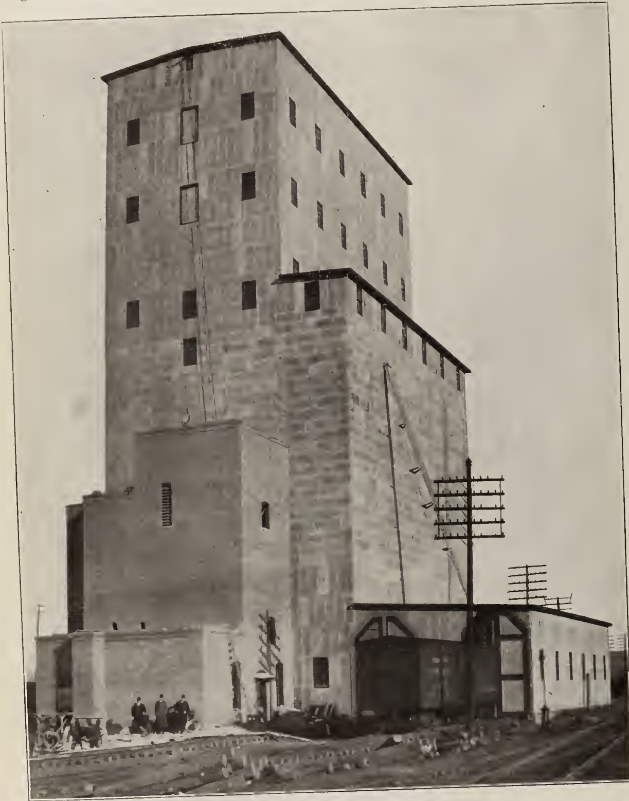
THE INTERSTATE GRAIN COMPANY'S ELEVATOR AT SIOUX CITY, IA.
