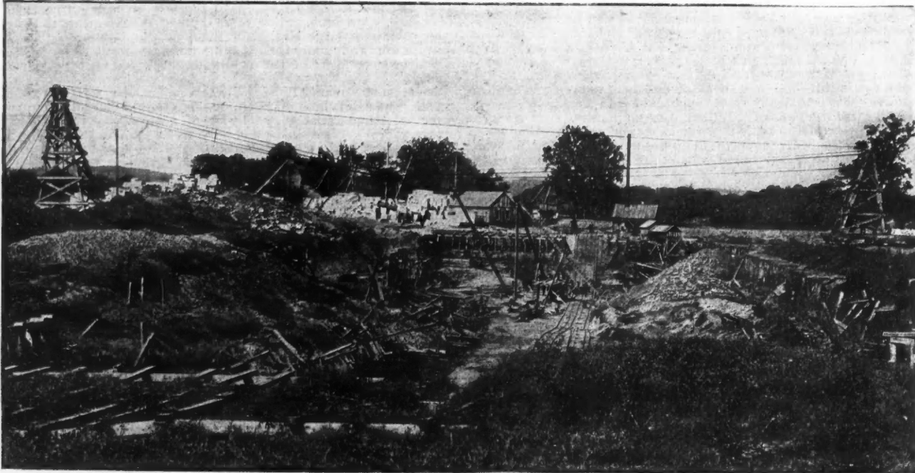
CABLEWAYS FOR THE PANAMA CANAL.
