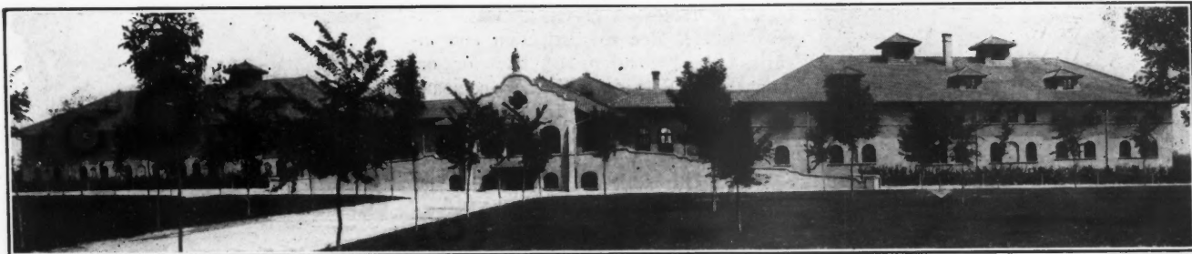
MAIN BUILDING, MINNEQUA HOSPITAL, PUEBLO, COLORADO
