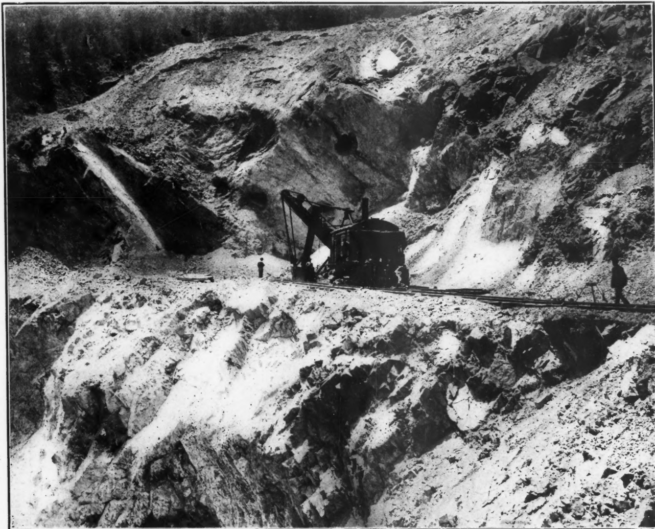
STEAM SHOVEL, UTAH COPPER COMPANY
