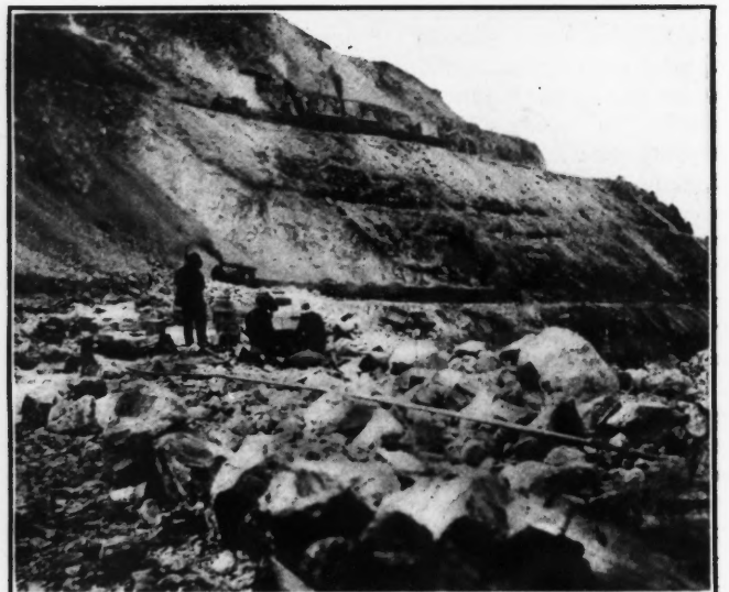
CHARGING DEEP BLAST HOLES, BOSTON CONSOLIDATED
