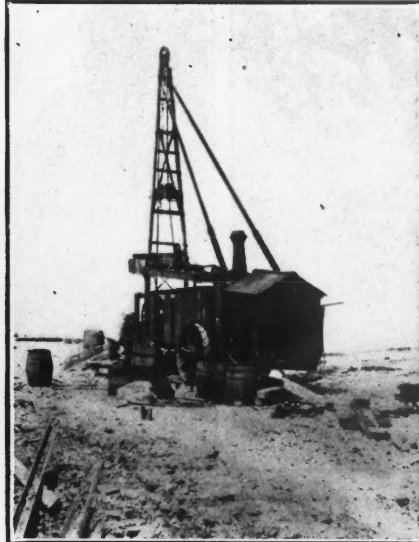
KEYSTONE DRILLING RIG, BOSTON CONSOLIDATED
