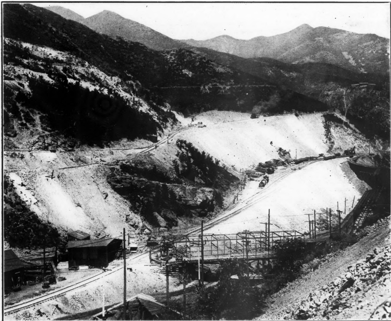
LOWER WESTERN PORTION OF THE UTAH COPPER COMPANY
