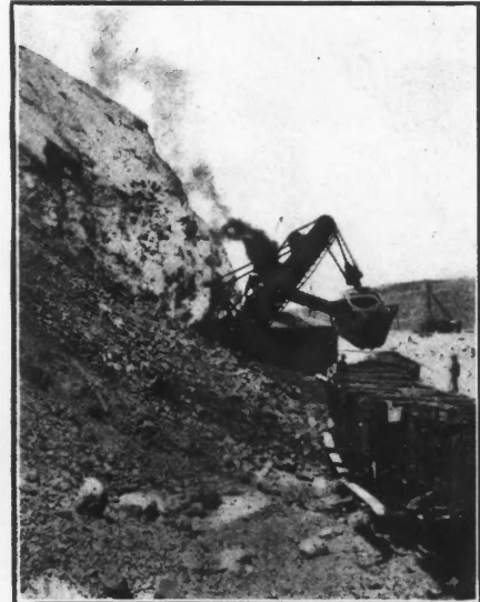
STEAM SHOVELS IN OPERATION, BOSTON CONSOLIDATED
