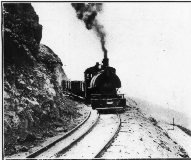
ORE TRAIN, BOSTON CONSOLIDATED
