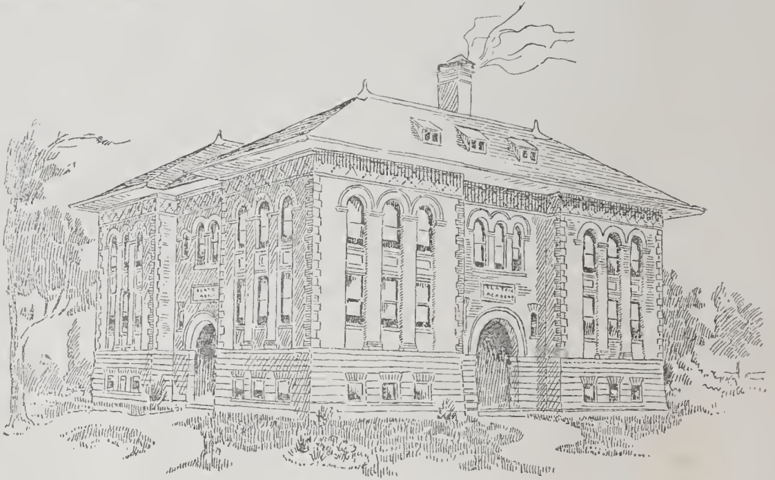
NEW BUILDING AT SLATER, JUST COMPLETED.
