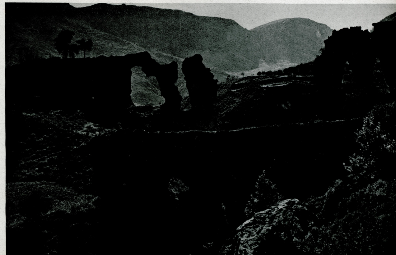
The Defne aqueduct
