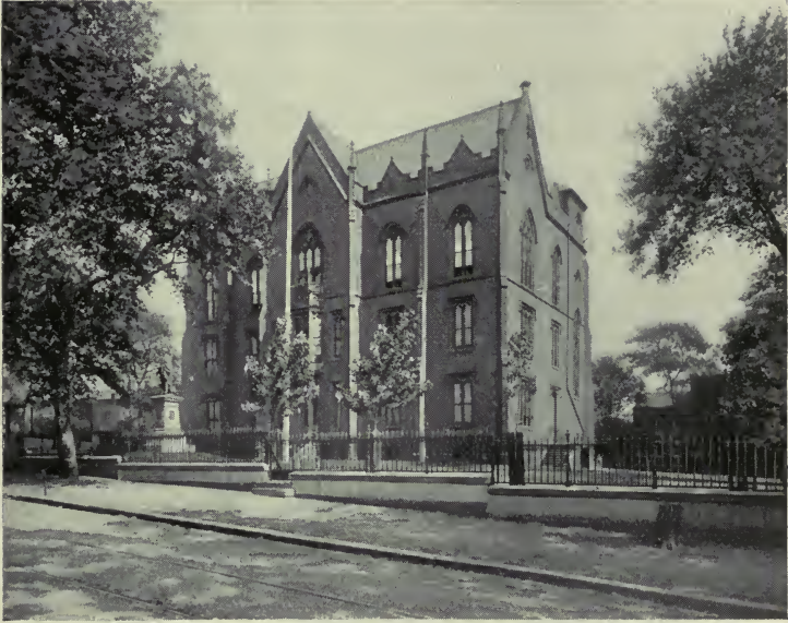
WOODWARD HIGH SCHOOL, Franklin and Abigail Streets, Between Sycamore and Broadway ; Erected 1854-5-67-80; Cost $73,037 ; 14 Rooms, Seats 582 Pupils; A. M. Van Dyke, Principal. (137)
