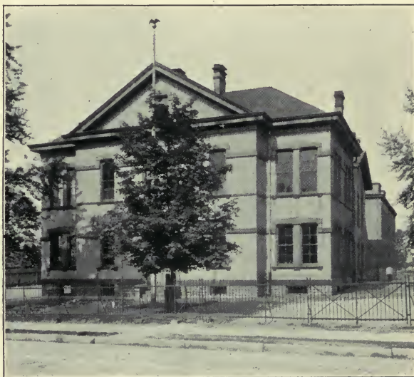
THE JOSEPH H. HOFFMAN SCHOOL, Formerly Nineteenth District; Erected, 1860-71-81-89; 19 rooms; Cost, $56,643; John A. Heizer, Principal; John Schwaab, Trustee.
