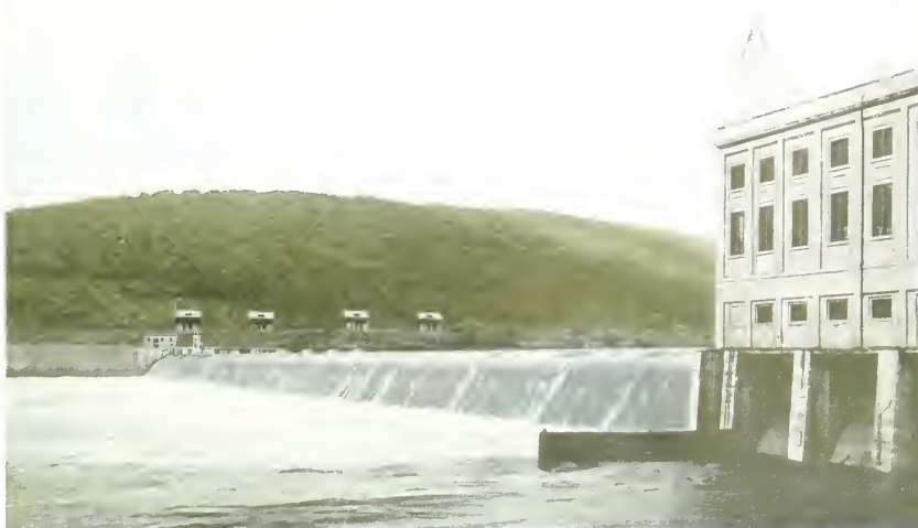
HALE'S BAR IMPROVEMENTS ON THE TENNESSEE RIVER NEAR CHATTANOOGA
