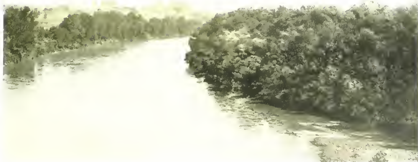
SITE OF DAM NUMBER ONE (FOR NAVIGATION ONLY) FROM FLORENCE BRIDGE.
