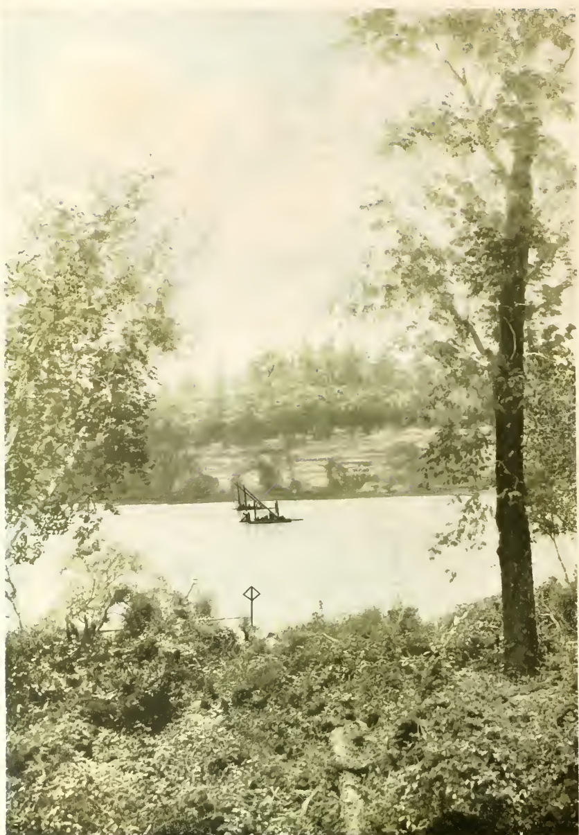
GOVERNMENT ENGINEERS DRILLING AT SITE OF DAM NUMBER TWO
