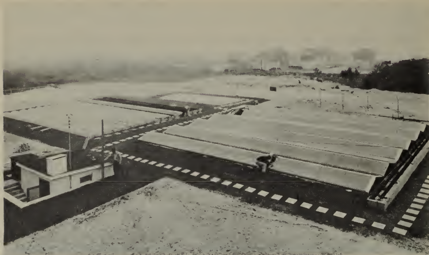
Using the sun's heat to desalt sea water. This solar research station south of Daytona Beach yields 500 gallons per day of fresh water.
