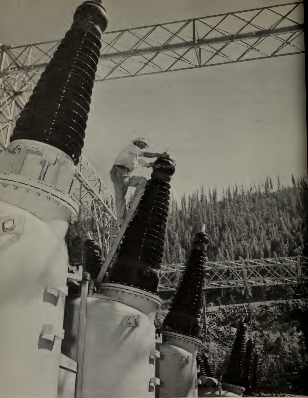
Power for western industrial expansion.—Hydroelectric power from Bureau of Reclamation projects plays a major role in the great postwar population and industrial expansion of the West. Revenues from power sales also are a major element in repayment of project construction costs. This workman is dwarfed by the huge bushings on the 230-kilovolt oil circuit breakers in the switchyard at the Hungry Horse powerplant in Montana.
