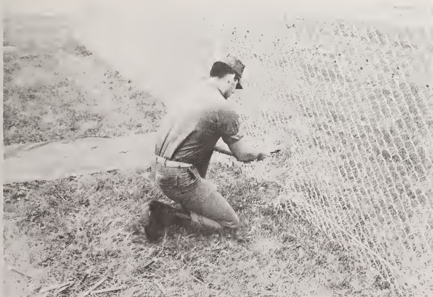
Figure 164. Cuts Being Made with Combination Fencing Tool; Test F1
