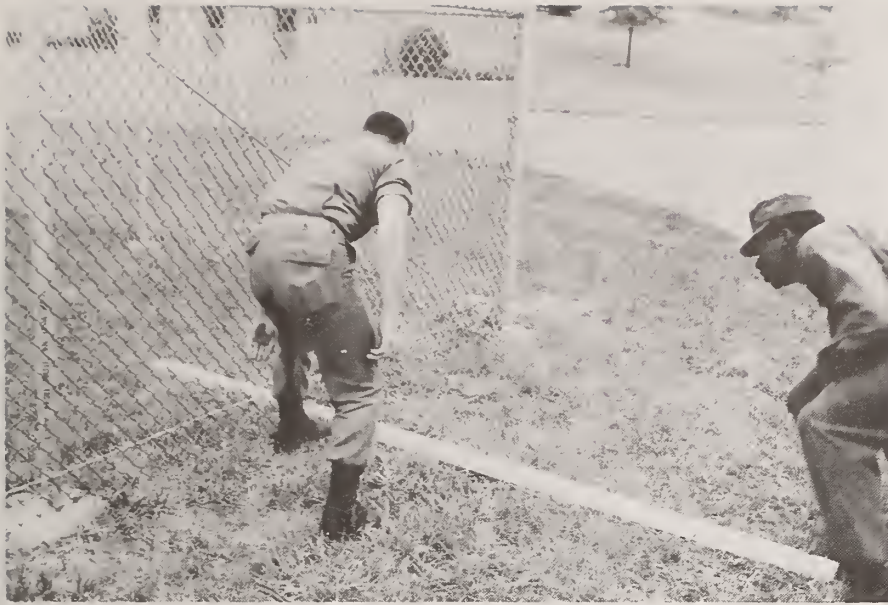
Figure 173. Placing 2 X 4 in Position; Test F2
