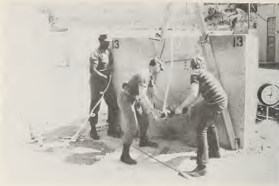
Figure 123. Test 13K. Two-man Operation of Suspended Battering Ram
