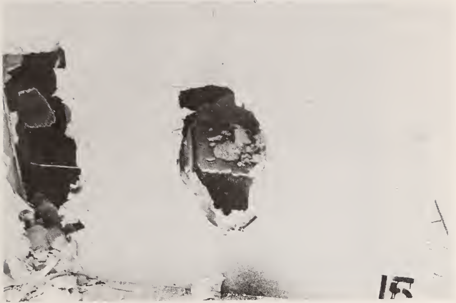
Figure 143. Test 15U. Final Size of Opening
