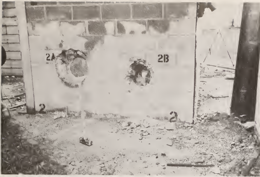
Figure 21. Breakthrough Hole after Numerous Blows; Test 2B
