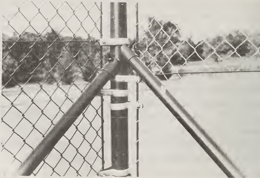
Figure 155. Fencing Using American Fittings To Attach Tensions Bars to Poles
