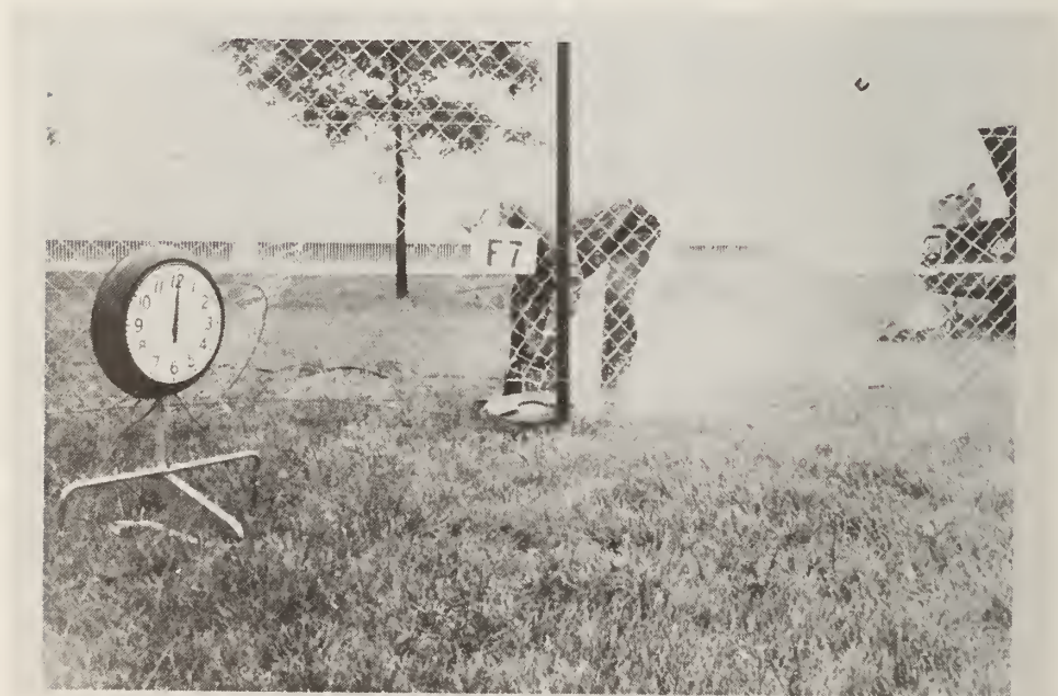
Figure 210. Cutting Metric Intermediate Post near Ground with Abrasive Wheel Saw; Test F7
