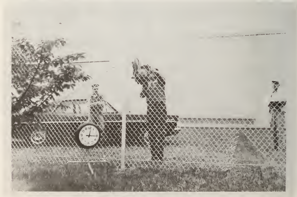
Figure 213. Cutting Full Height of Fabric with Abrasive Wheel Saw; Test F7
