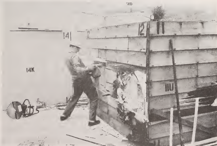
Figure 102. Cutting with Hubless Saw; Test 12
