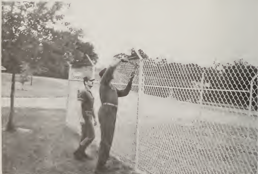
Figure 168. Cutting Wires which Attach Outriggers to Tops of Poles; Test F1
