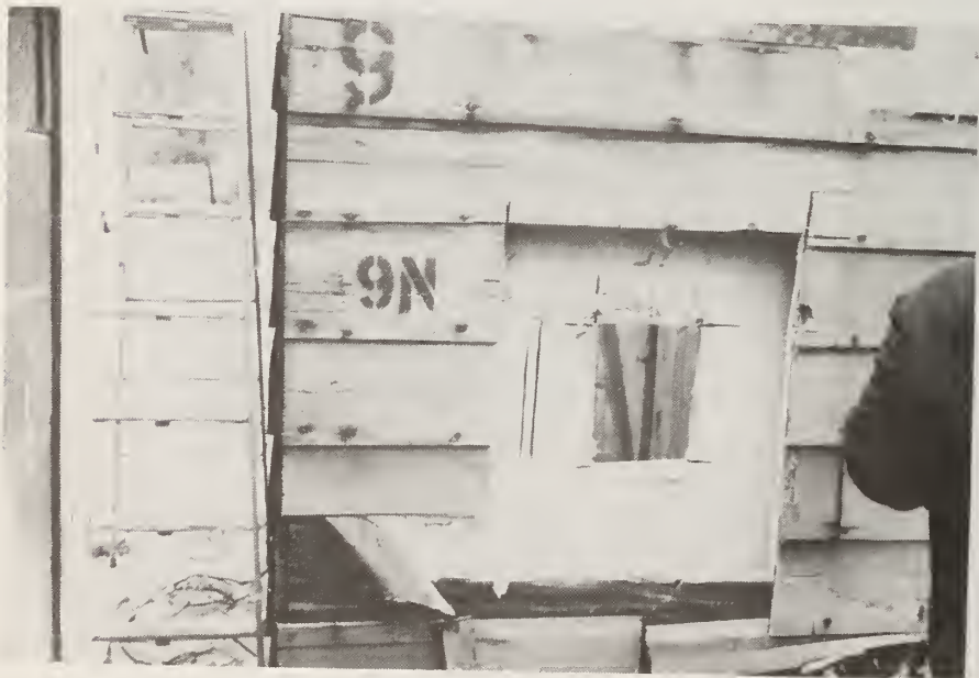
Figure 80. Test 9N. Completed Opening
