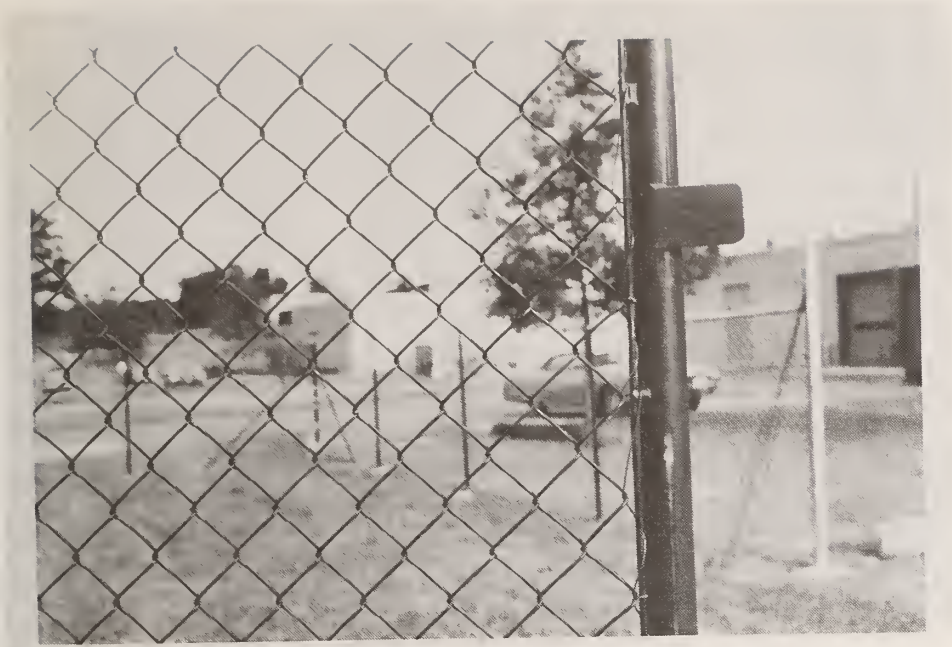
Figure 194. Details, Metric Fabric Attachment to Gate Frame; Test F4
