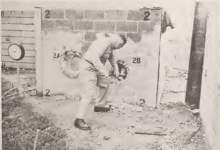
Figure 22. Enlarged Opening with 26-lb. Bar; Test 2B
