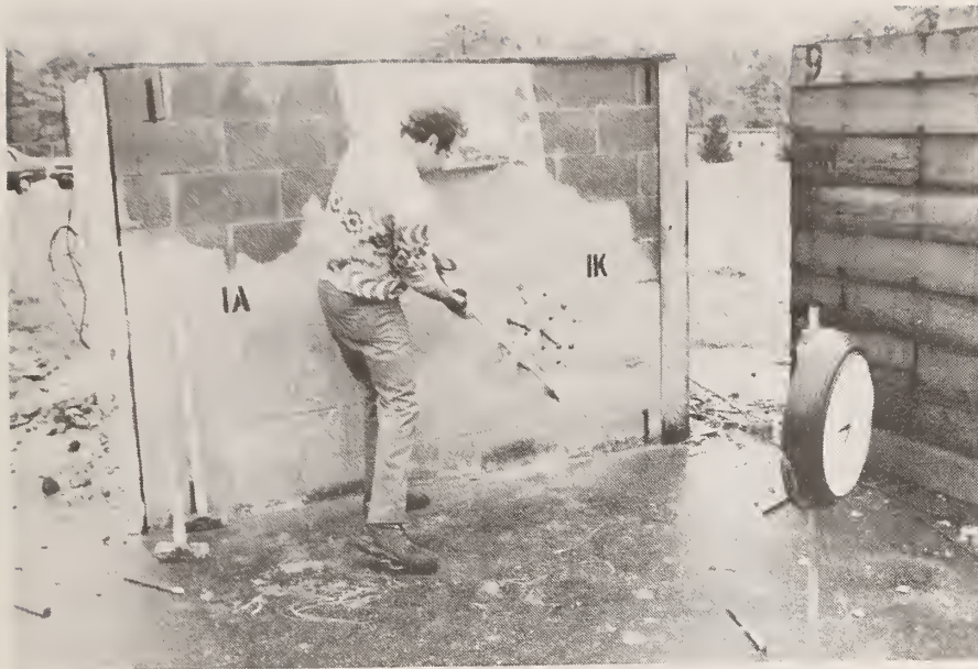
Figure 5. Spalling from Hole Pattern; Test 1K
