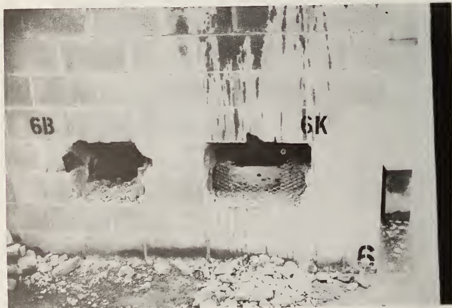
Figure 51. Opening Produced by 50-lb. Battering Ram and No. 14 Bolt Cutters; Test 6K
