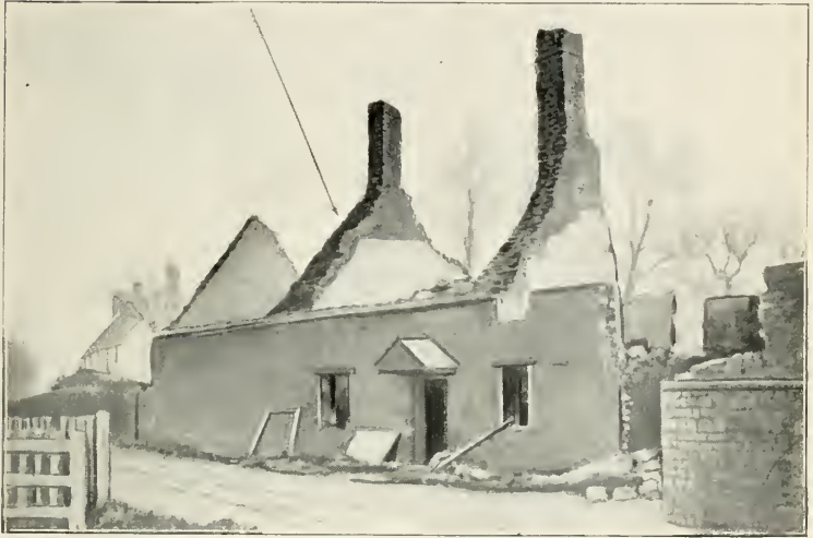
THE BURNT-OUT HOUSE OF THE SMITHS
