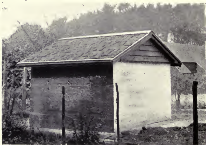
THE FRUIT-HOUSE COMPLETED WITH ROOF OF PEAT BLOCKS ON ROUGH BOARDING.
