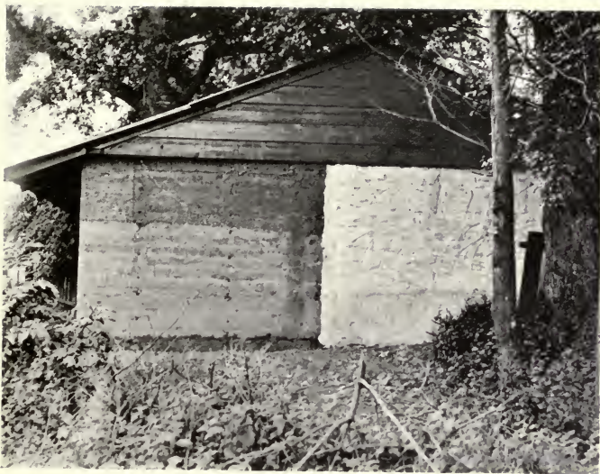
PISÉ WAGGON-HOUSE AT NEWLANDS CORNER. An experiment in rendering.
