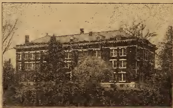
NEW HALL OF RESIDENCE
