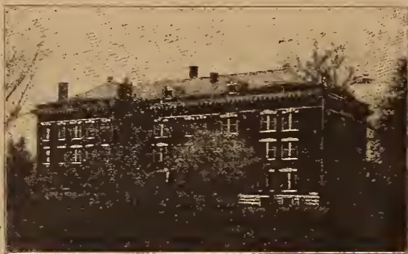
NEW HALL OF RESIDENCE
