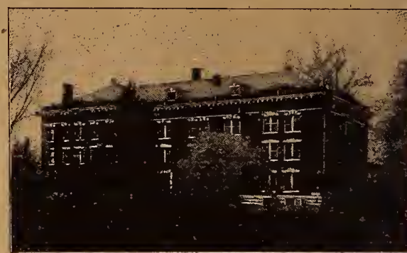
NEW HALL OF RESIDENCE
