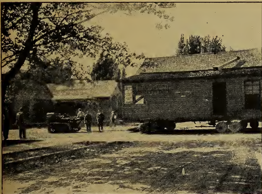
Here is a farm tractor that is pulling a house. The house weighs more than five tons. The building was moved ten blocks, a part of which was up a five per cent grade. The altitude of this Idaho town is 4,500 feet. This tractor will pull three 14-inch plows. It is one of several medium-priced tractors that will plow eight acres in a ten-hour day at a small expense
