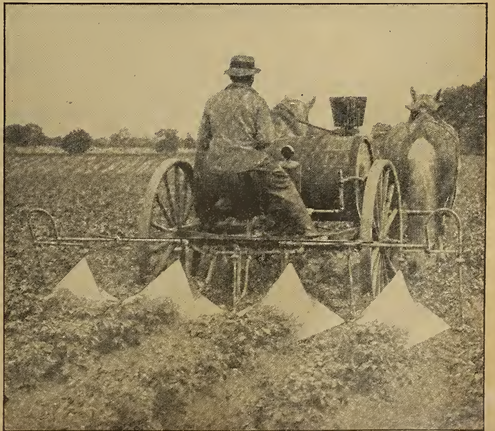
I N HANDLING large orchards the man without a power sprayer can't give the pests "knock-out drops" fast enough to put them out of business, and keep them out. This is a four-man power outfit, one man to drive and attend the machinery, and three men to spray. A crew of this size can handle 125 acres of orchard, and apply more than 100 wagon loads of spray mixture a week if necessary. A pressure of 200 to 300 pounds to the square inch can be maintained
