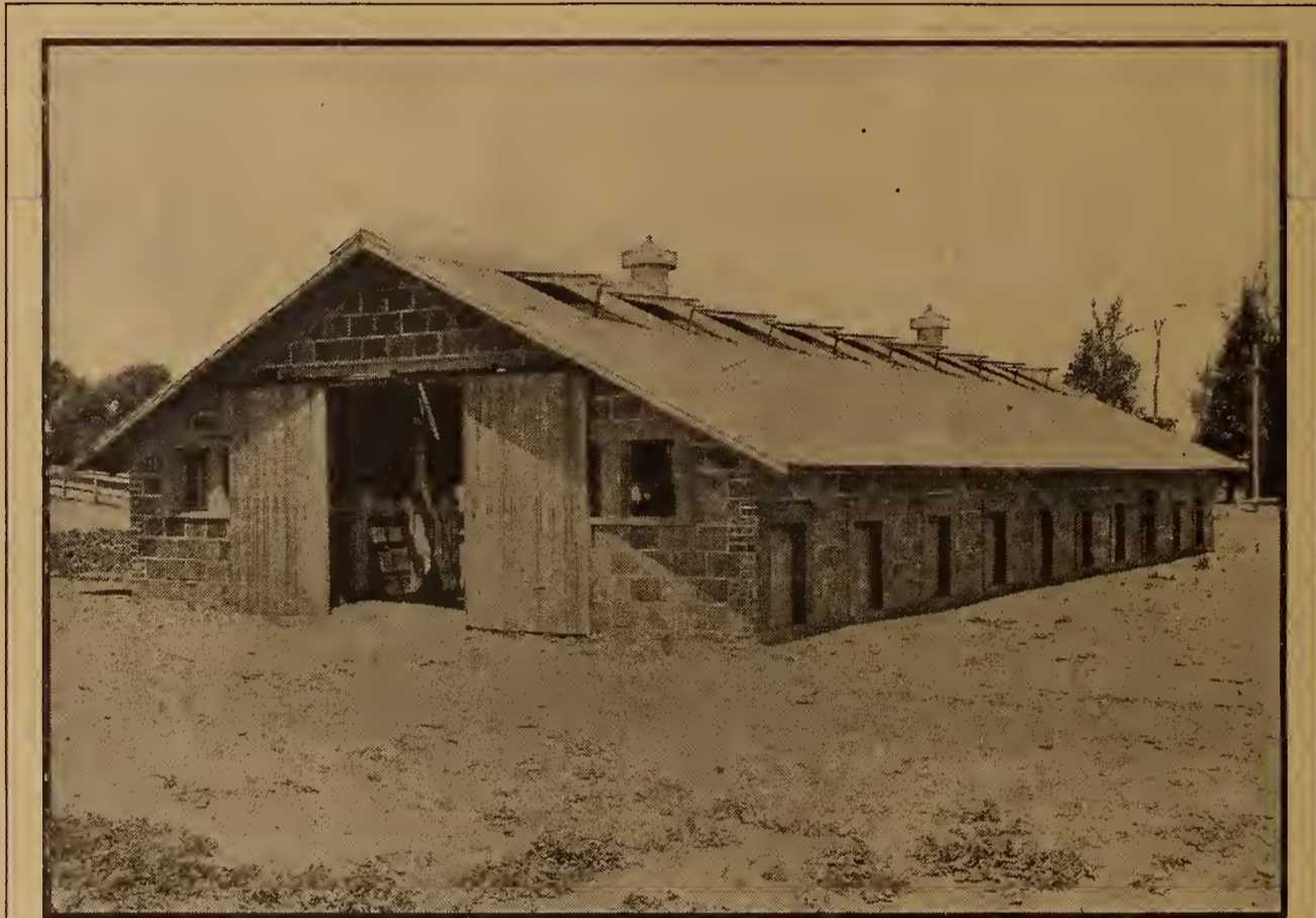
The Iowa sunlit hog house costs from $25 to $40 a pen, depending upon the grade of materials used and the amount of equipment installed. It differs from other houses chiefly in its method of lighting
