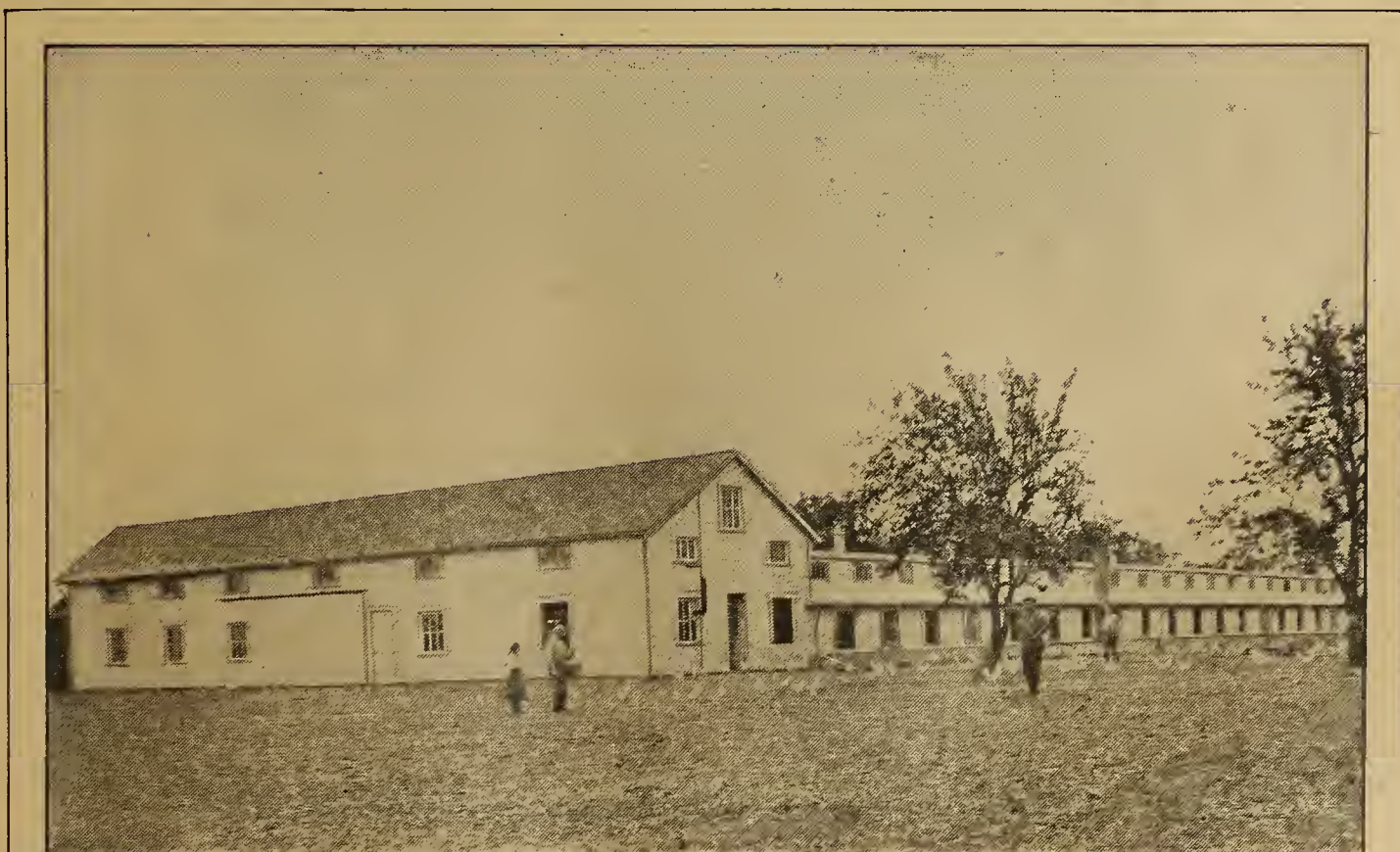
Twelve hundred Leghorn hens use the egg-laying house of the Dayton plant. The egg-laying house is the right wing of this building. It is 200 feet long, and has a concrete floor and foundation
