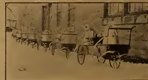
One of the newest things in mechanical milking. Each truck contains a complete milking-machine outfit operated by a small engine
