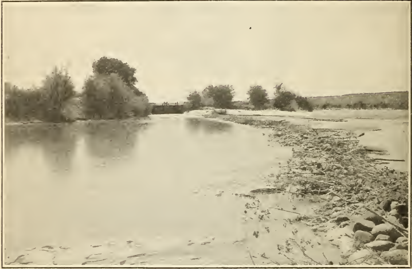
FIG. 4.—Temporary dam and headgate of irrigating canal, Gila River.
