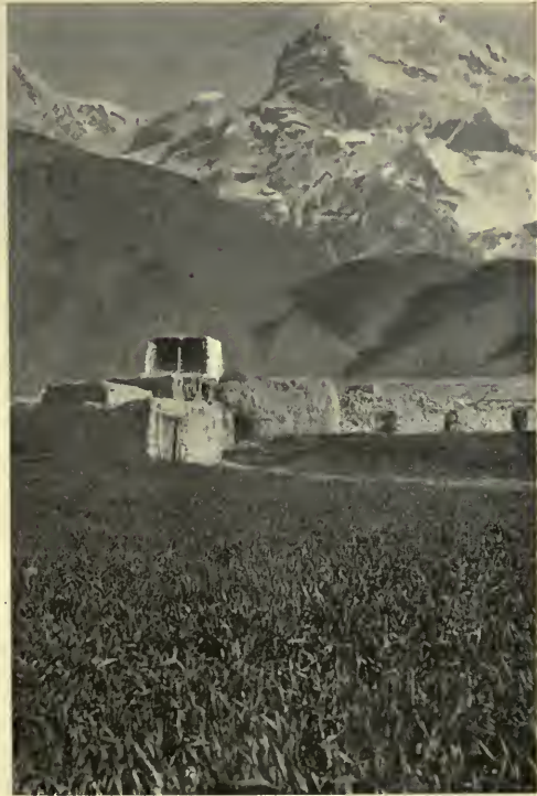
THE HOUSE OF THE MIMBASHI AT ROSHOR
