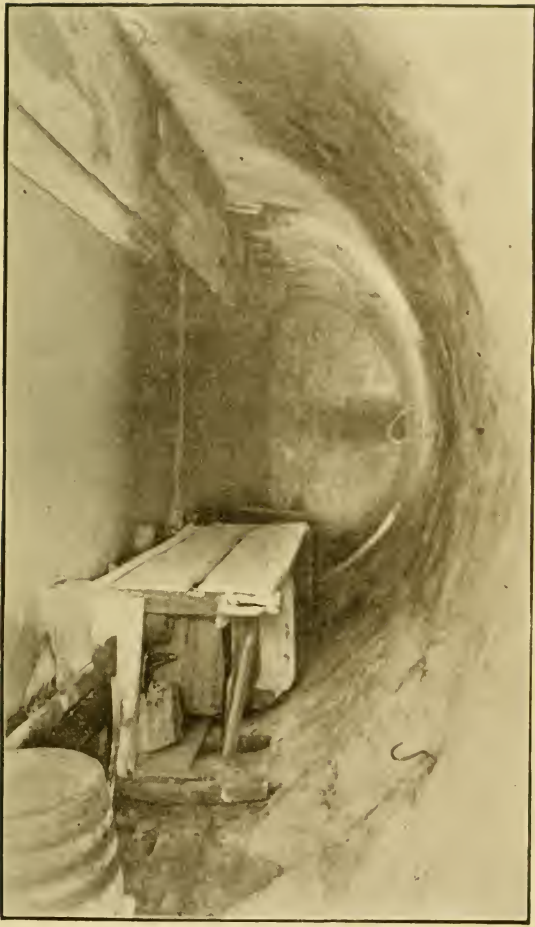
UNDERGROUND IN CRESSAP'S FORT
