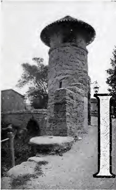
MEMORIAL BRIDGE, MILFORD, CONN.
