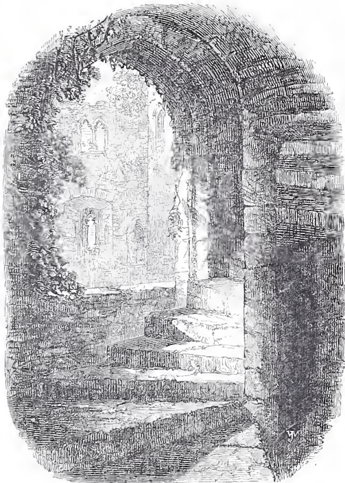
STAIRCASE IN GWENT TOWER.
