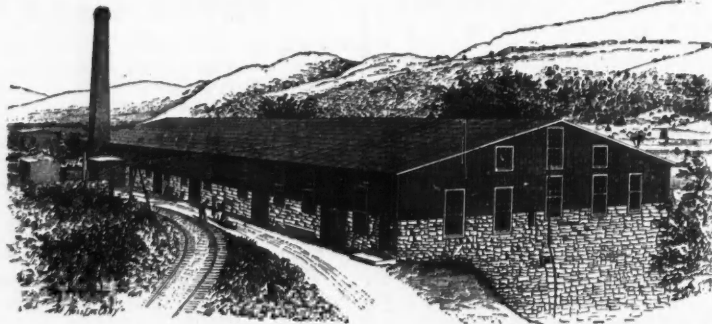
The above illustration is taken direct from a photograph, and shows the exterior of a Marble Mill, designed and built by us for The True Blue Marble Co., at Rutland, Vt. The building is built entirely of Iron and Marble, the foundations being of marble; all the supporting members of the building are made of Iron. The sides of the building are made, for a height of 10 ft., of refuse marble blocks, the balance of the covering of the sides being of corrugated iron.
