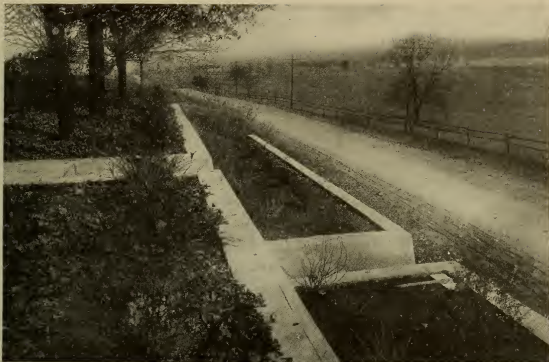
39. Concrete terrace or retaining wall. Showing a pleasing method of breaking up a very steep slope.
