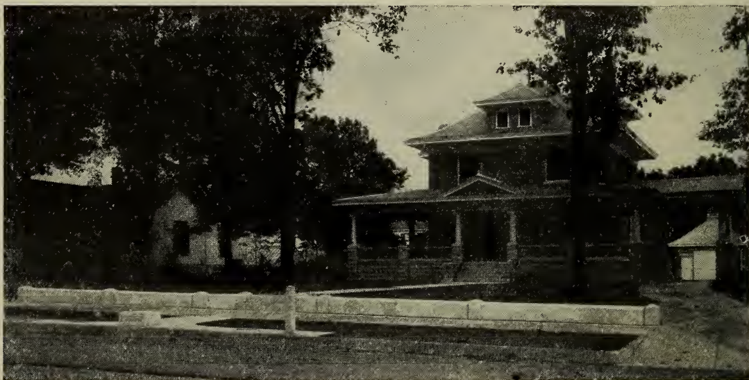
35. Horse-block and hitching-post of concrete, with small retaining wall in background. Only home-made forms are required in this construction.
