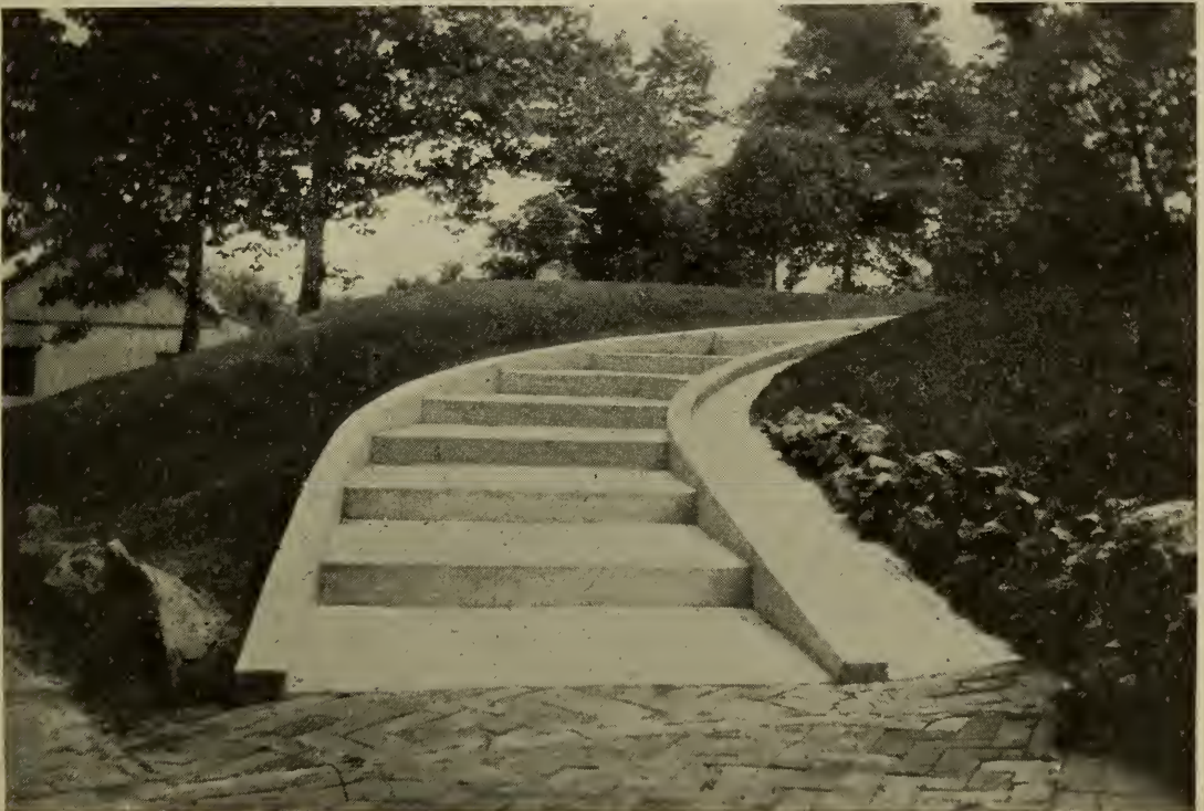
10. The outdoor step of concrete offers, in the making, a very pleasing method of entrance to the home.
