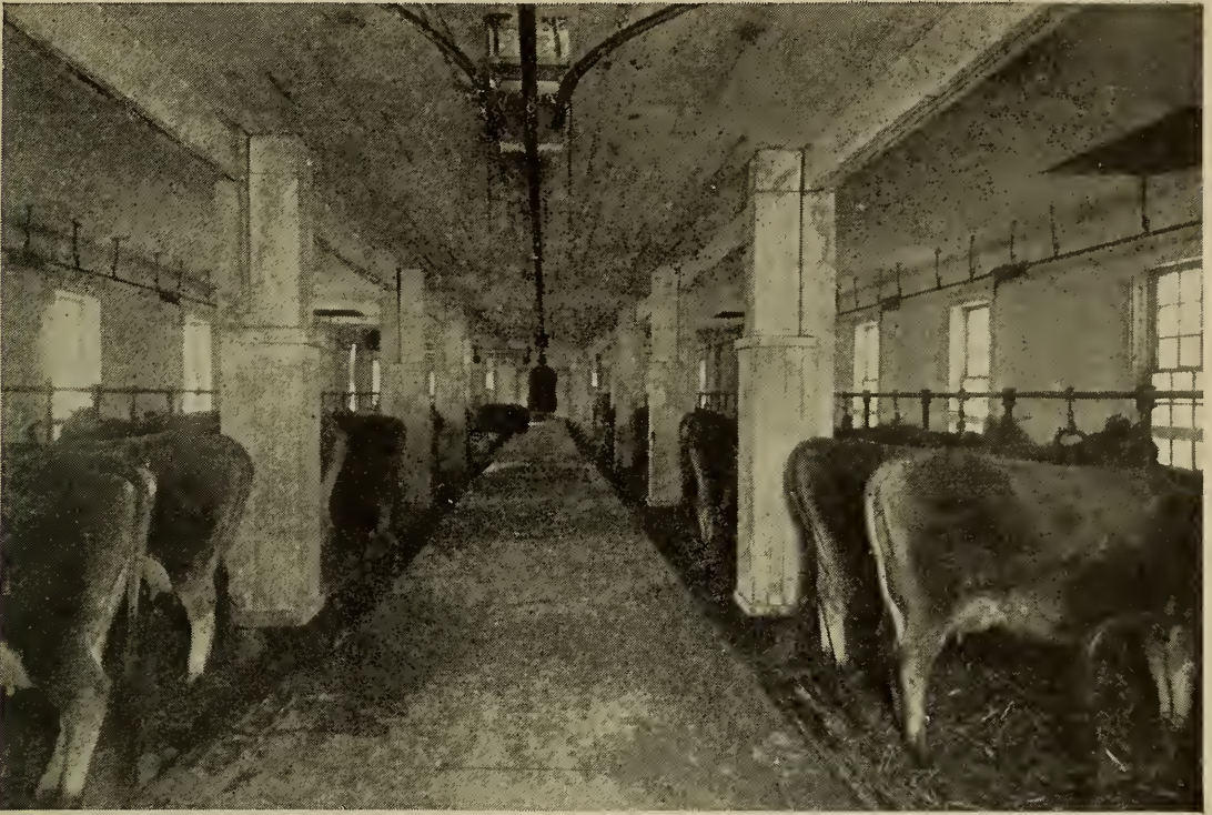
56. Interior view of large stock barn, showing method of facing stock toward windows. The carrier suspended from the ceiling simplifies bedding and cleaning.
