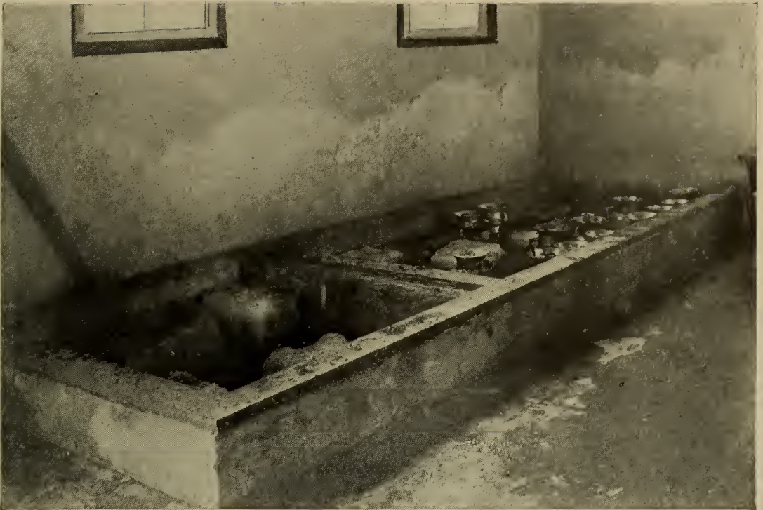
68. Milk-cooling tank in modern dairy establishment—construction of same shown on next page. A bracket overhead would simplify handling of cans.
