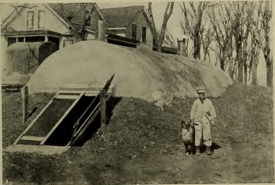
45. An outdoor storage or root cellar is a comfort, luxury and economy—it is also inexpensive to build.
