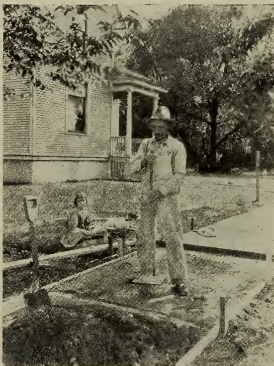
26. Method of tamping concrete in sidewalk work.
