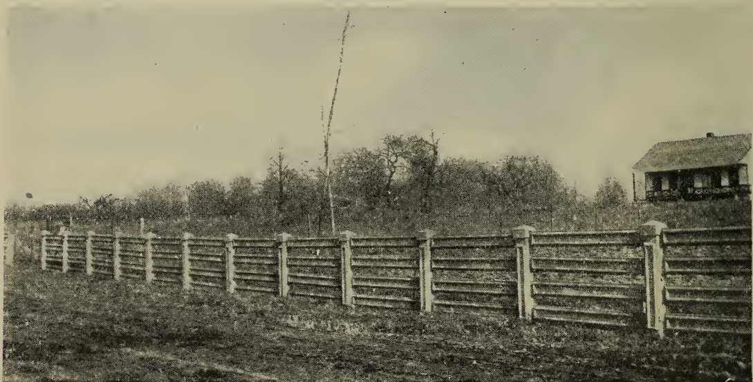
30. This type of fence, though more costly than one of posts and wire, has the advantage of being absolutely permanent.
