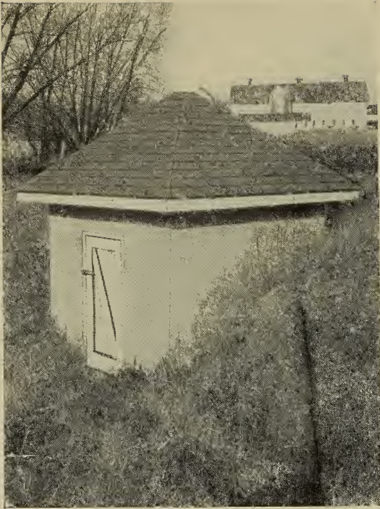
85. A concrete ram house is simple to build and affords permanent protection to the ram.
