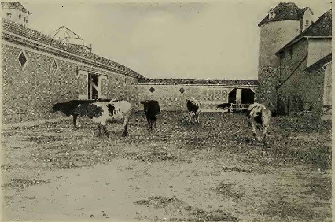
61. A concrete feeding floor that saves both food and stock. This floor can be thoroughly and quickly cleaned.
