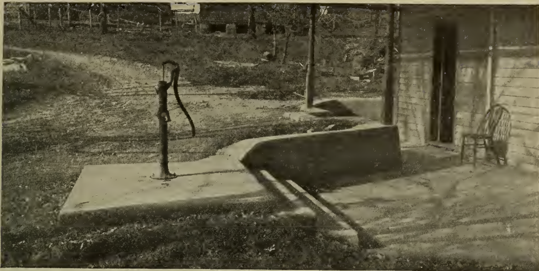
18. Concrete well platforms keep the water pure and the health of the family in good shape. If properly built they improve the appearance of the place.
