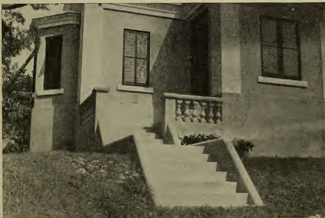
7. Besides being utilitarian, the concrete porch is capable of very pleasing appearance. Design of house and contour of ground decide whether angles or curves be used.
