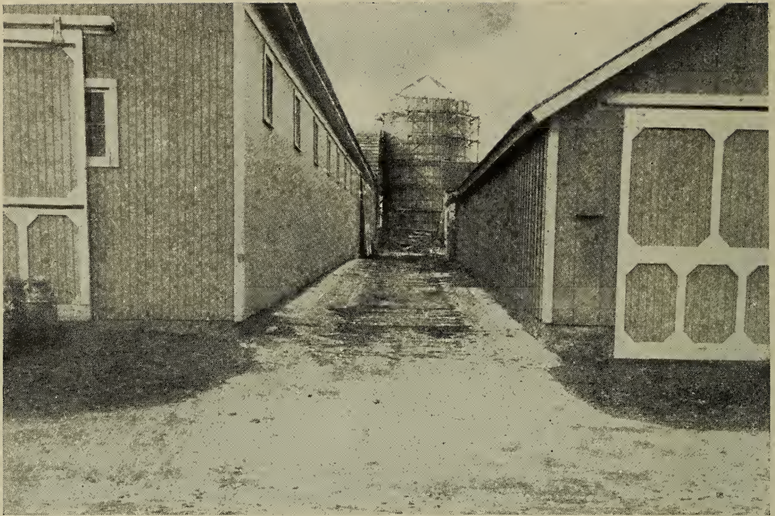
63. Concrete alleyway and feeding floor. A slight slope toward the center keeps the water away from the foundations.
