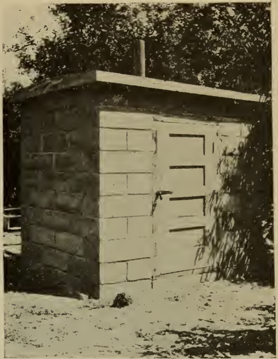
86. Such a smoke-house may be built of blocks, metal lath, or monolithic construction. If concrete, it's permanent.
