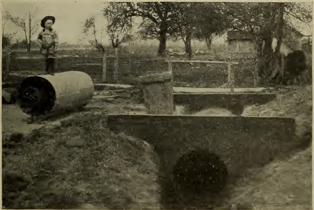
82. Commercial forms for building culverts. These forms are collapsible, rendering them easy to remove.
