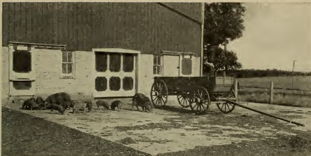
62. Small concrete feeding floor. It also affords an easy entrance to barn in bad weather. This is a good investment for both comfort and economy.
