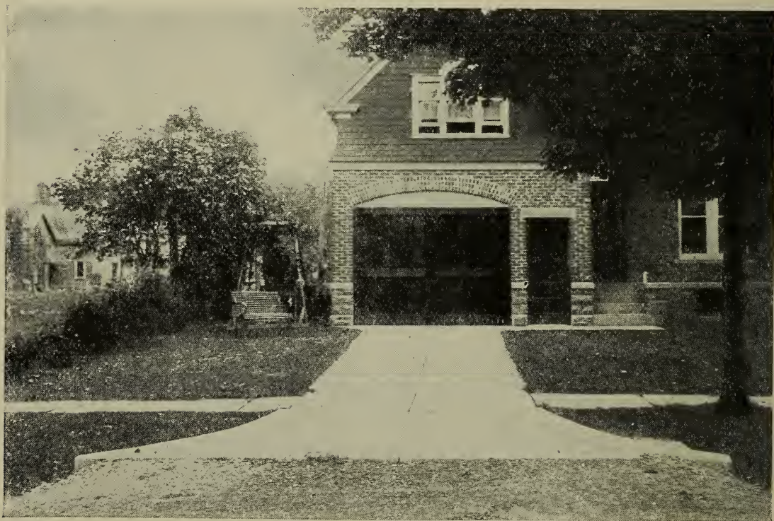
23. A concrete driveway helps keep lawn and garage neat in appearance. A slight slope should be provided to take care of drainage.
