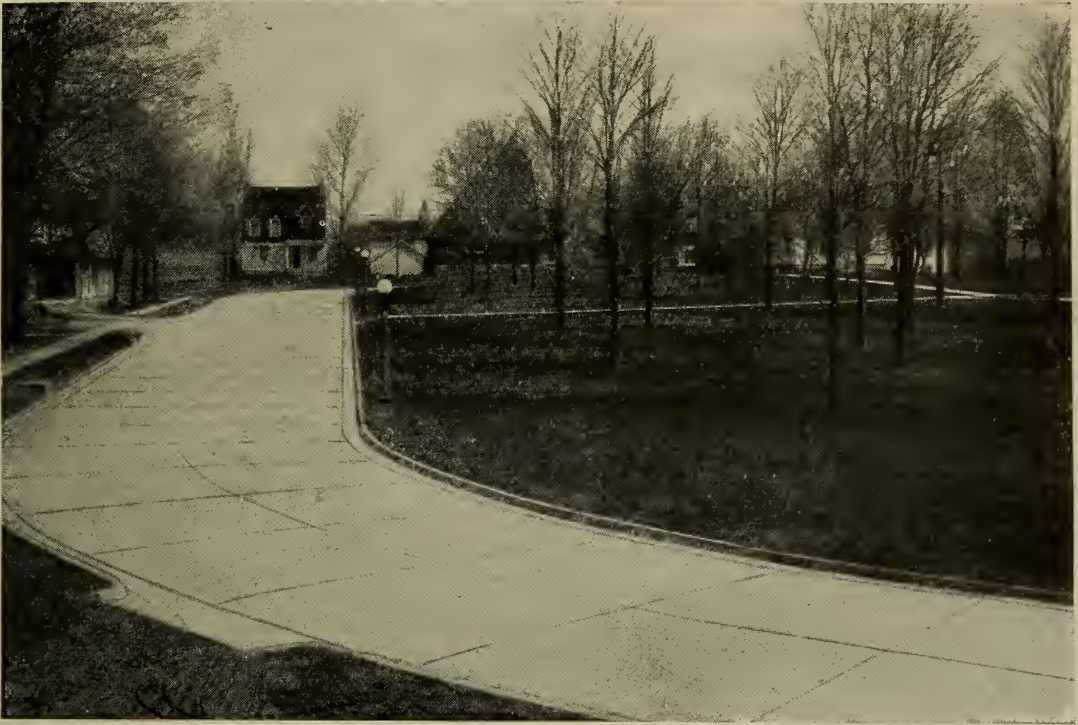
24. Through large estates and parkways the concrete driveway is becoming a favorite because of its self-maintenance.
