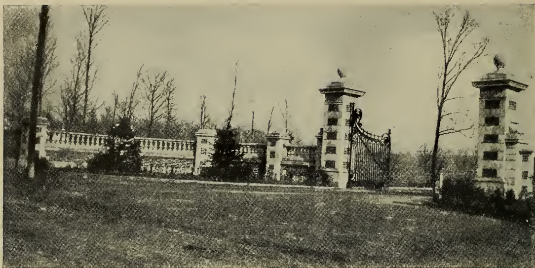
34. A combination concrete and brick post, showing a rather unusual treatment. This method of handling is suitable for large country estates.
