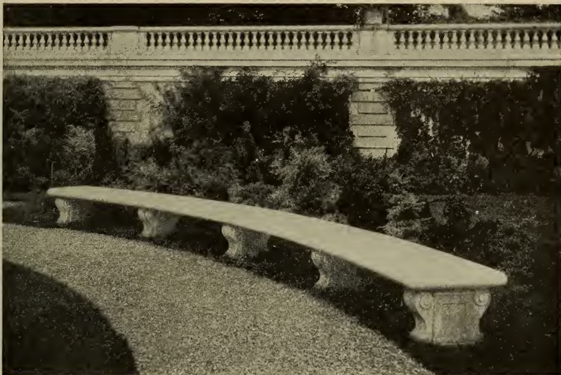
27 and 28. Two very simple types of concrete benches, simply slabs placed upon uprights which in turn rest upon concrete bases.
