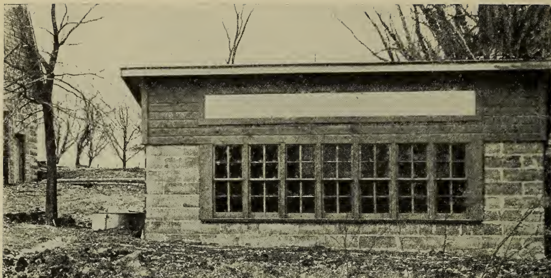
77. A muslin curtain above the windows gives constant access to fresh air. The windows themselves hinge in against the roof.
