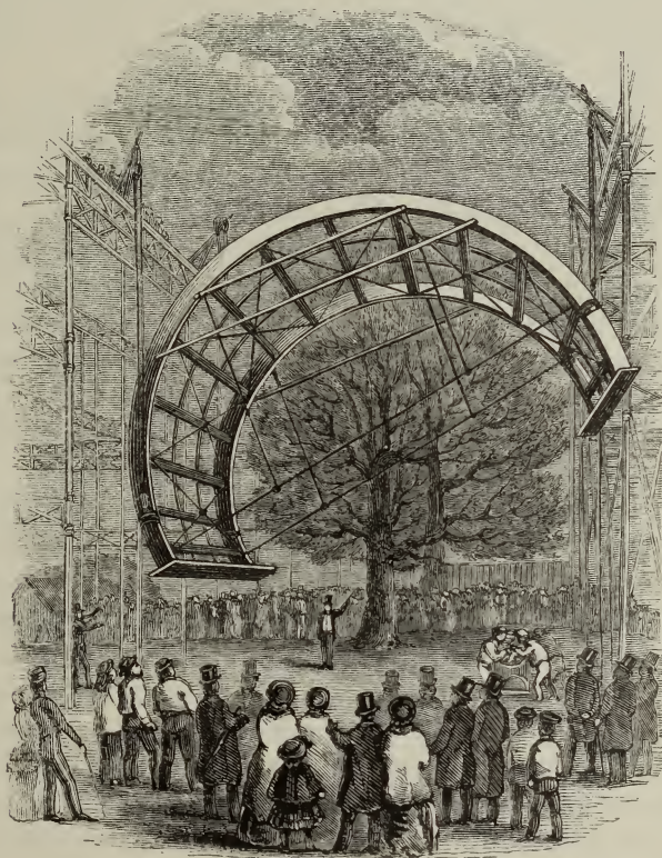
RAISING THE TRANSEPT-RIBS.
