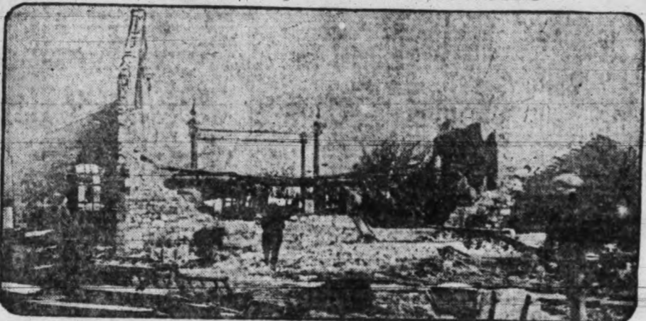
The latest form of violence in Ireland is the systematic destruction of municipal waterworks by the followers of De Valera. Here is all that is left of the municipal waterworks in historic Athlone after a rebel bomb had exploded.
