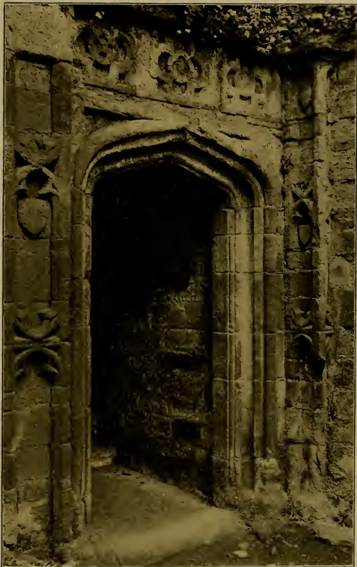
THE DOORWAY OF THE KEEP, LUDLOW CASTLE.
