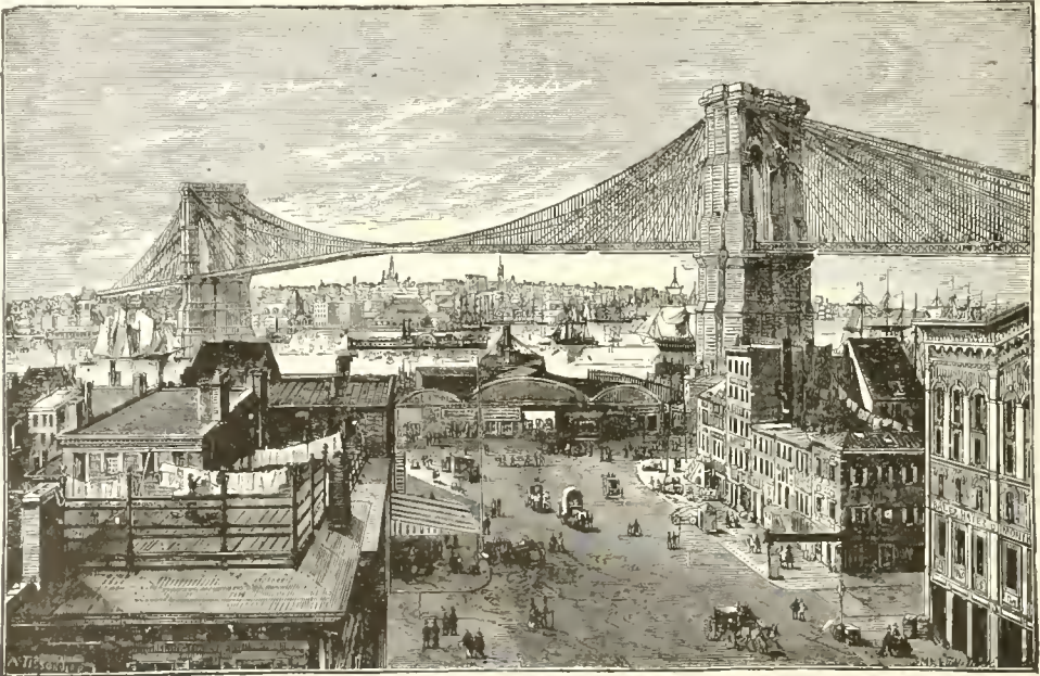
EAST RIVER BRIDGE.
