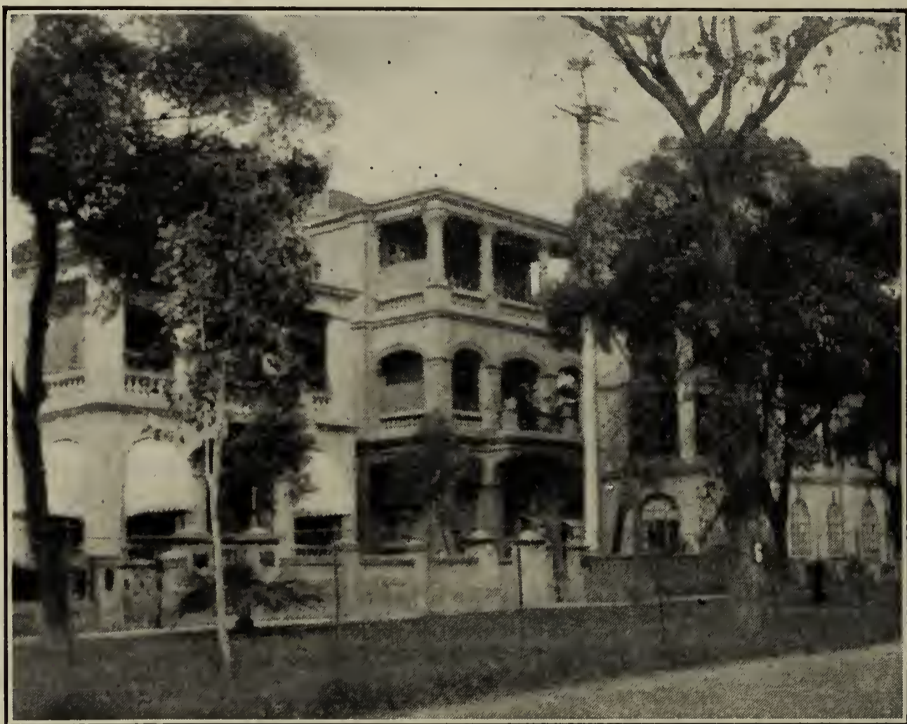
FIG. 16.—American consulate general, Canton. The United States has had a consular representative at Canton since 1784
