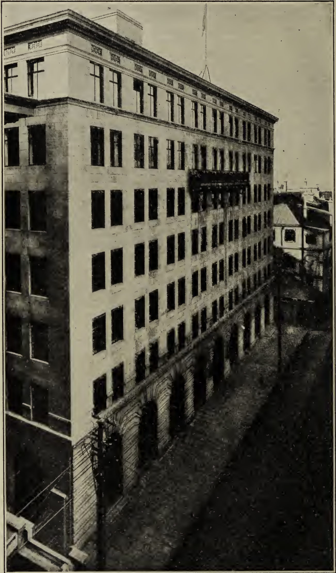
FIG. 18.—Robert Dollar Building, Shanghai, in which are located offices of American commercial attaché
