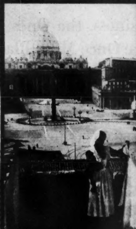
ROME, from a housetop, Camillo Cianfarra has charge of U. P. service here.
