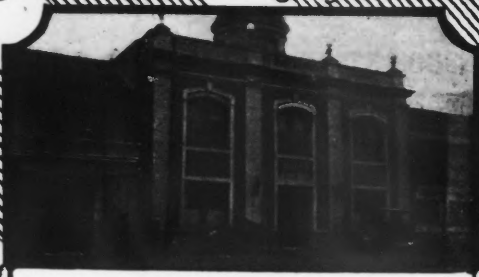
Japan Advertiser building, TOKYO (under reconstruction).
