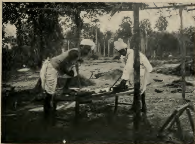
Carpenters at work on the new Asylum, Ramachandrapuram.
