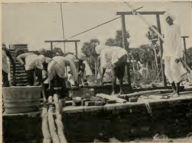
Bricklayers building the new Asylum, Ramachandrapuram.
