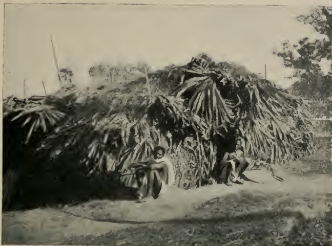
Temporary Huts for lepers. Ramachandrapuram.
