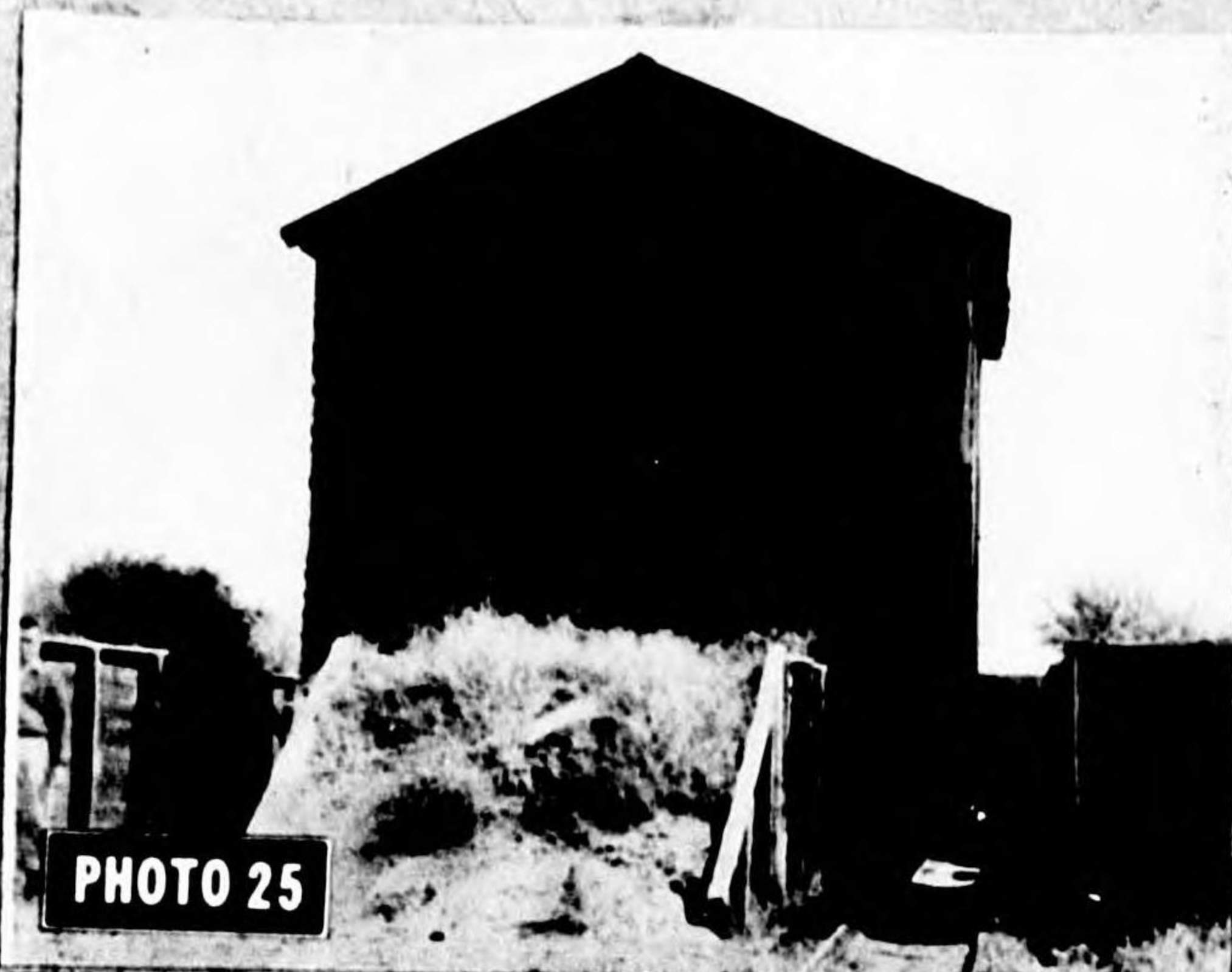
Mobile house covering radar, Kawasaki.
