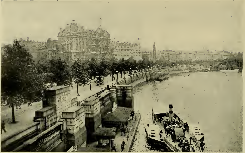
Thames Embankment, from Hungerford Bridge.
