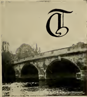
Bridge at Henley.
