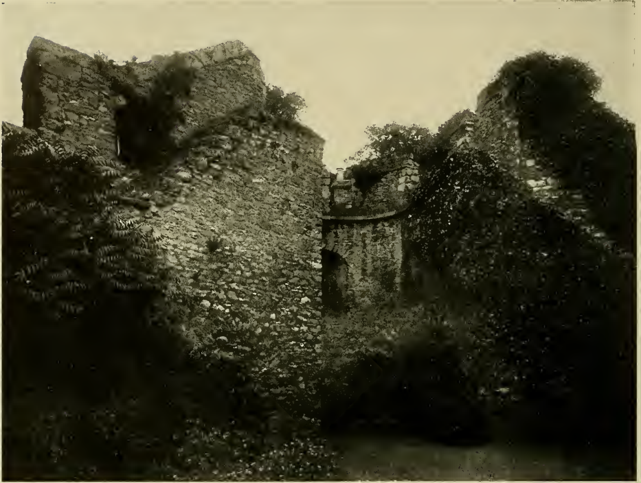
Old City Wall at New College, Oxford.
