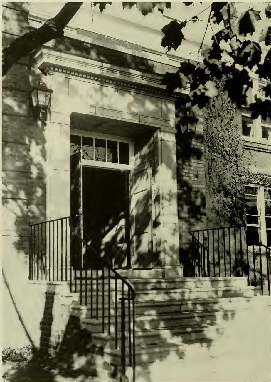
Remodeled Entrance to North Spencer
