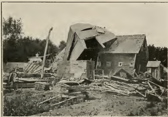
FIG. 14. Effects of tornado, Watertown, S. D., June 23, 1914.
