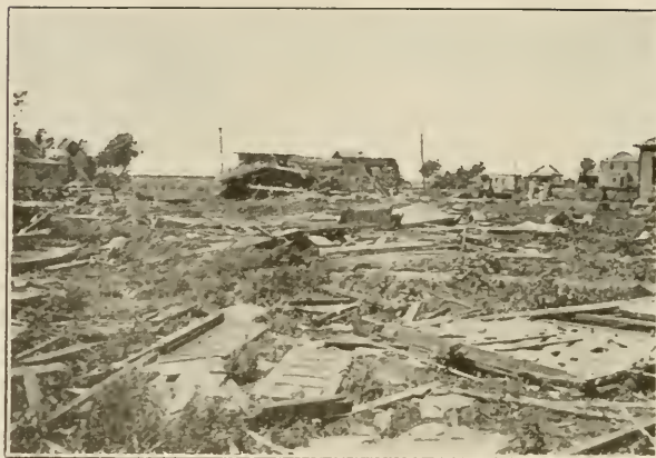
FIG. 11. General view of wreckage where destruction was greatest. Watertown, S. D., June 23, 1914.
