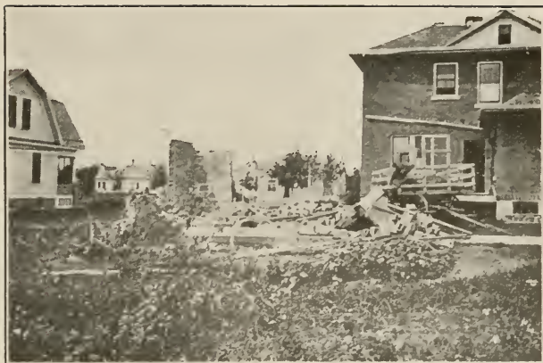
FIG. 9. Collapse of hollow tile structure. Watertown, S. D., June 23, 1914.
