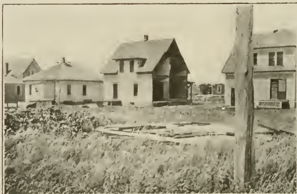
FIG. 4. House with end blown outward.
