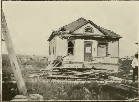
FIG. 15. The tornado passed to the left of this house moving toward the reader. The porch was torn away and deposited in the rear of the house. Watertown, S. D., June 23, 1914.
