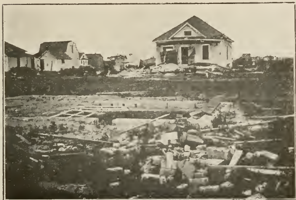
Fig. 10. The house from the foundation in the foreground was carried bodily across the street and then dropped to the earth and broken to bits. Wreckage may be seen in front of cottage on the right.
