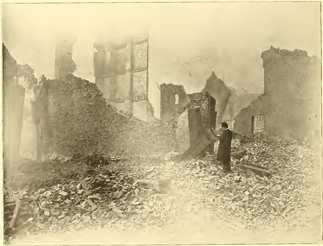
Looking northwest from German and Light streets, bonded warehouses and wholesale whiskey district. All buildings totally destroyed.
