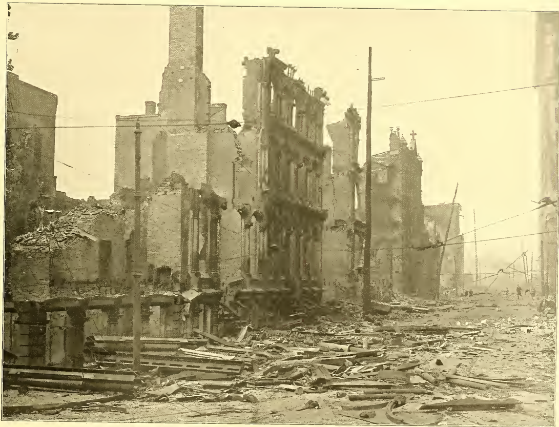
View from corner of German and South streets looking Southwest.
