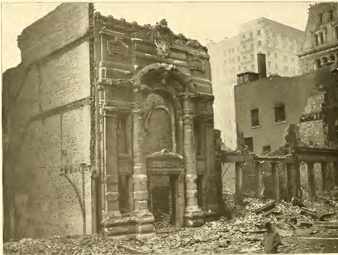
Banking house of Hambleton & Co. looking towards Baltimore & Ohio Central building.
