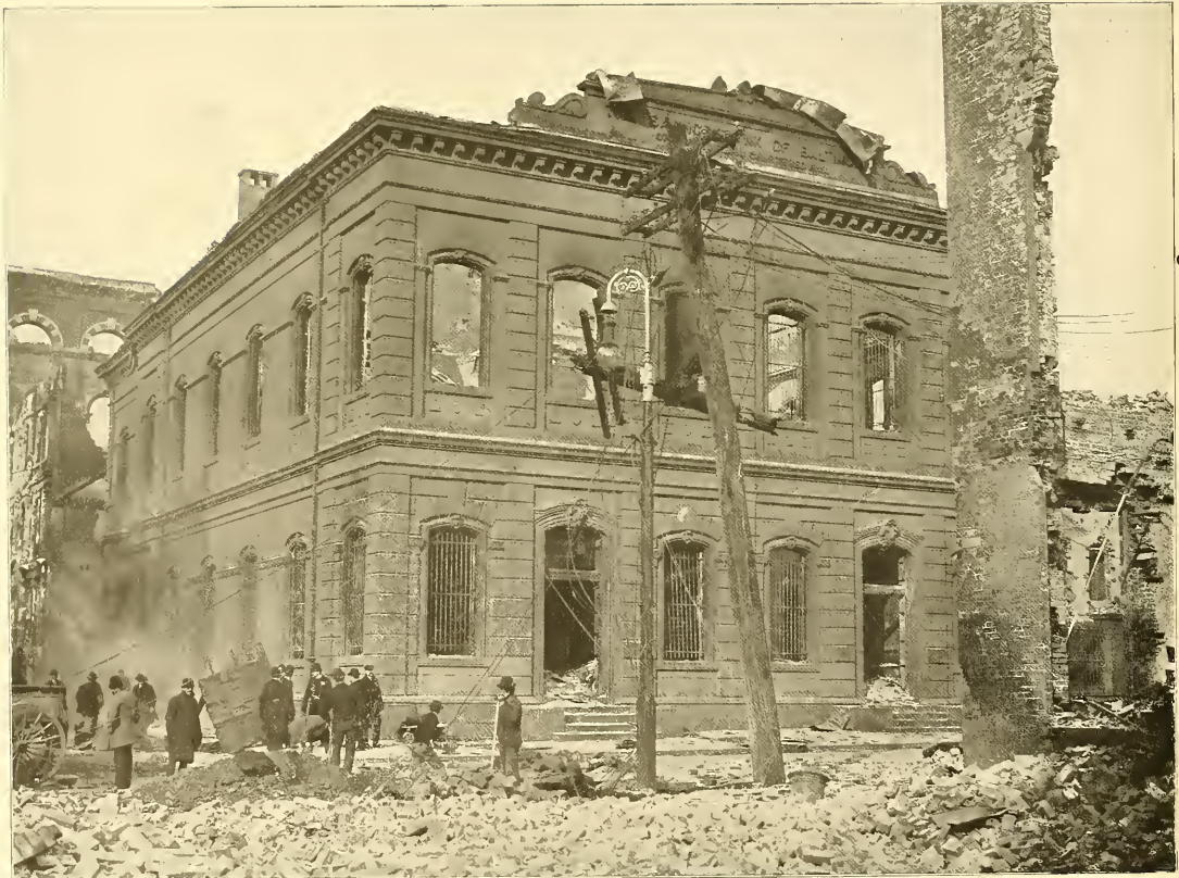
Savings Bank of Baltimore. Nothing left of building except the outside walls.
