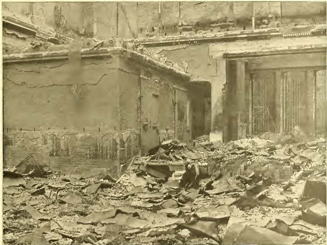
Interior view First National Bank, nothing left but the large vaults, which were proof against the intense heat, all securities were found in perfect condition.
