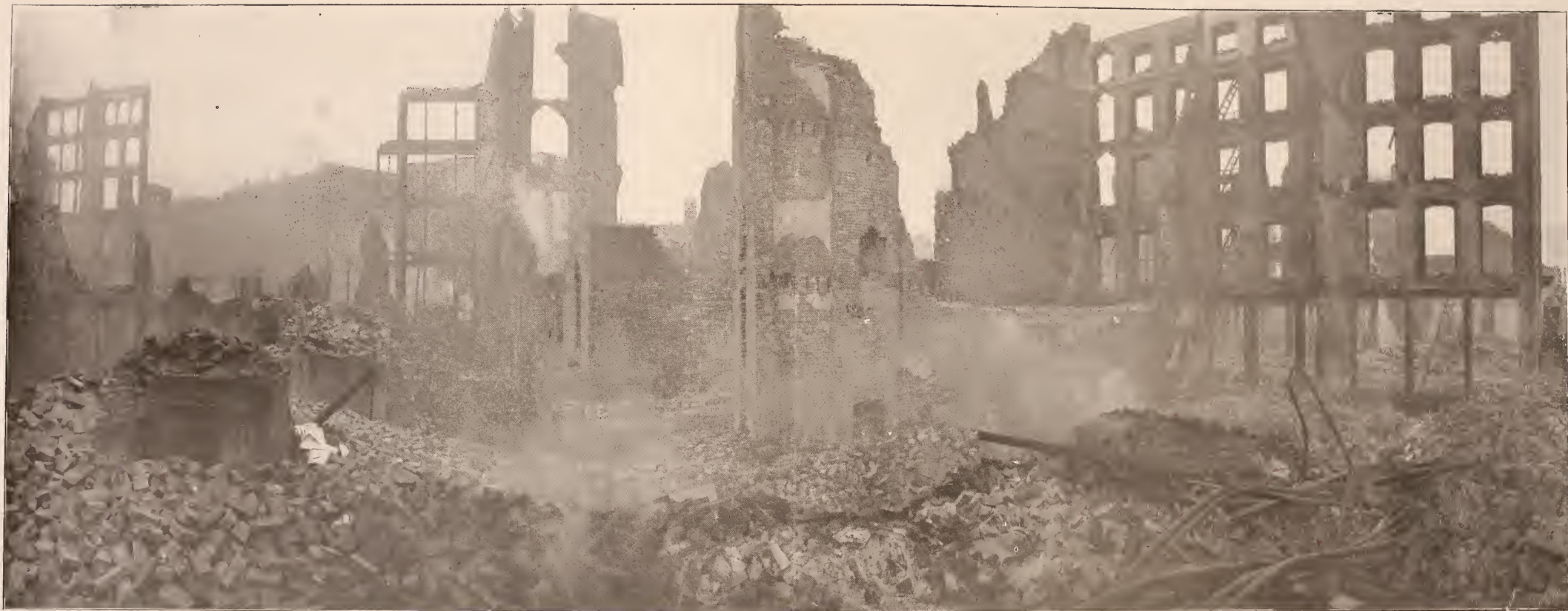
View from German and Hanover streets, wholesale business district, all buildings and contents totally destroyed for several blocks.
