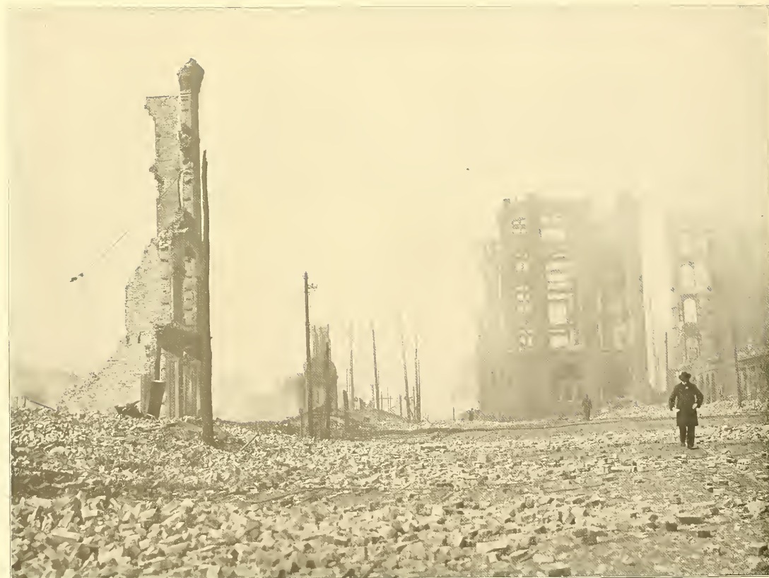
General view from corner of South Lombard street looking West, showing several very fine office and bank buildings completely destroyed.
