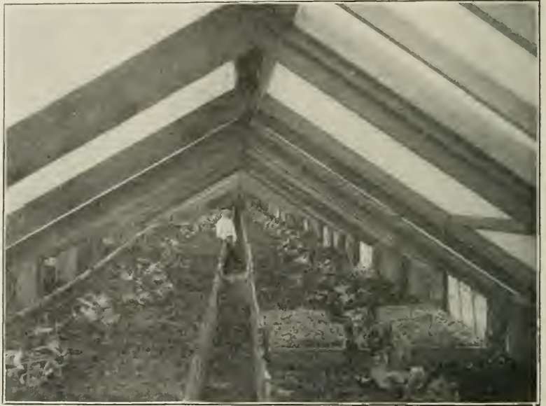
Interior of Cucumber House After Plants Are Set
